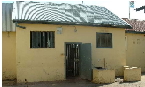
Enlarged kitchen addition from internal courtyard
