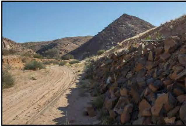
Figure 9. Rocks have been packed on the lower hillslope to limit erosion and the watercourse is used as a farm road during dry periods.
