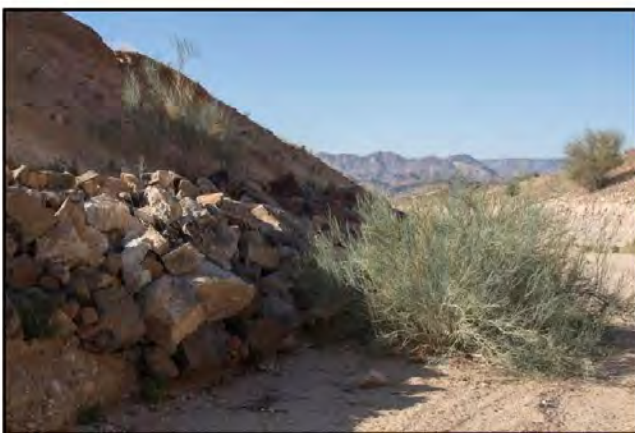
Figure 8. Rocks stabilised by wire cages (gabions) at the foot of a hill slope, to prevent erosion. The grey-green plant is Sisyndite sparteae , typical of seasonal dry watercourses in this arid environment.
