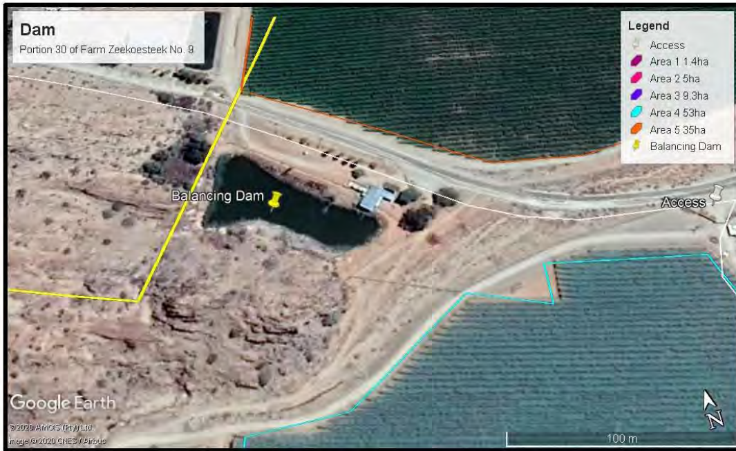
Figure 2: Locality of the dam
