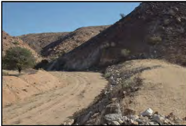
Figure 13. The diversion embankment packed with rocks to prevent erosion.
