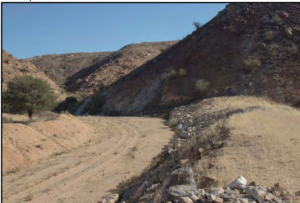
Figure 16: The diversion embankment packed with rocks to prevent erosion.
