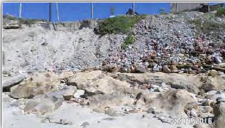
Figure 5: Arniston harbour embankment.
