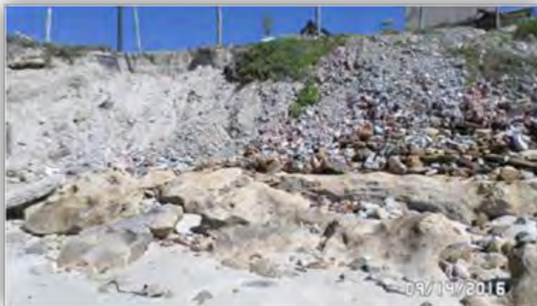
Figure 5: Arniston harbour embankment.
