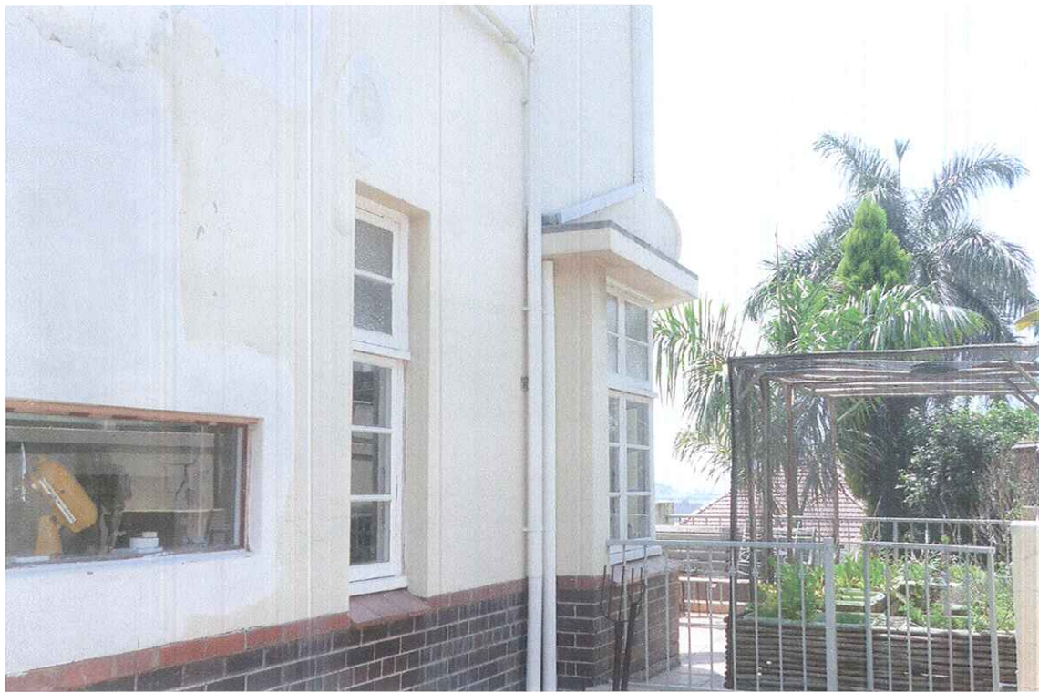
PORTION OF SOUTH FACADE
