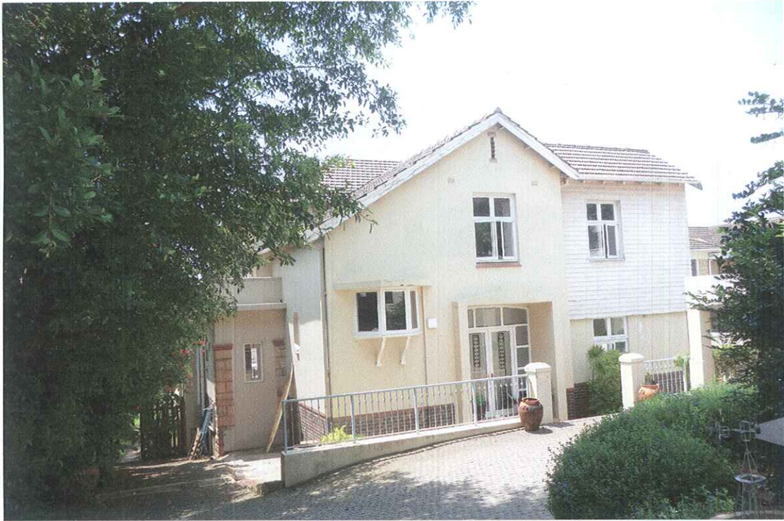
WEST FACADE (FACING ROAD)
