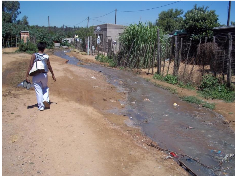
Figure 4: Raw human sewerage was flowing down the street along the proposed alignment of the new sewer collector line.
