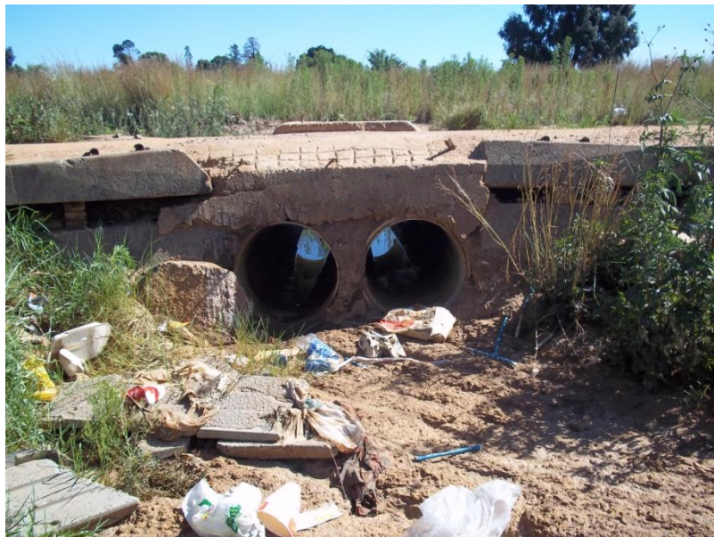
Figure 7: The canal flows under a low level bridge before entering a series of dilapidated ponds or dams.
