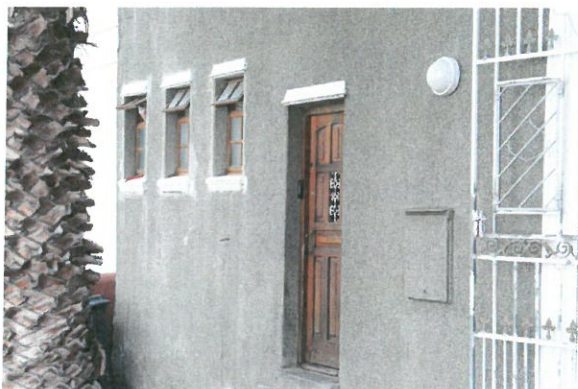
Doorway and bathroom windows adjacent to entrance
