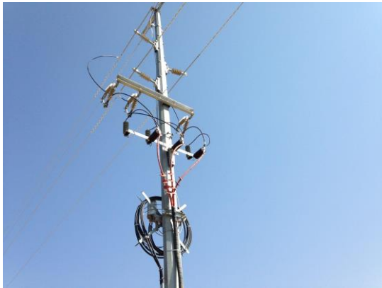
Figure 8: Cable termination on an overhead line. The structure offers several possibilities for places for nests to be built, either by crows or by Sociable Weavers.
