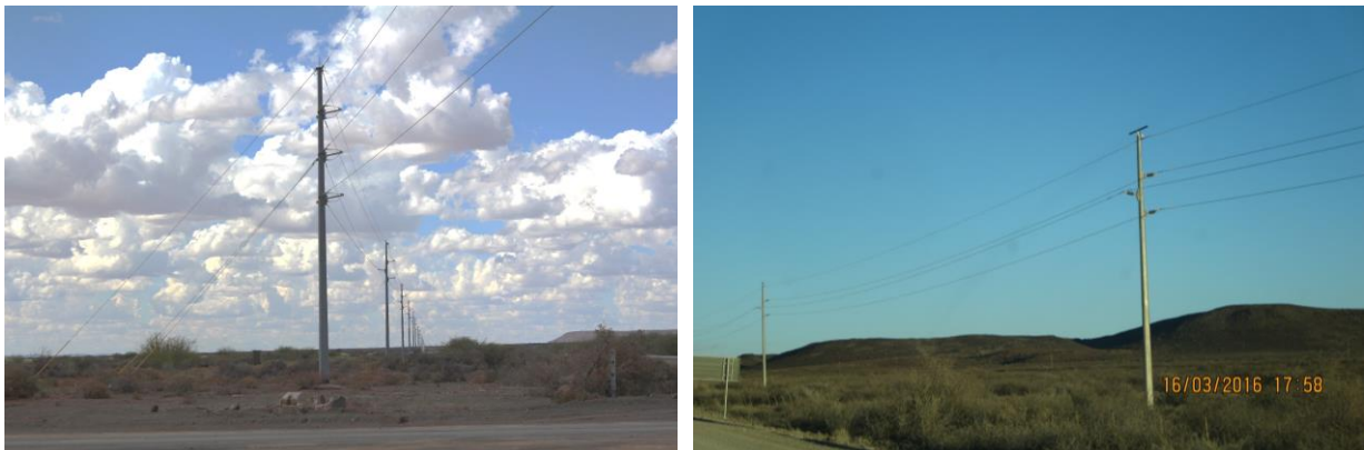
Figure 5: Two different designs of powerline poles in the SKA area.
