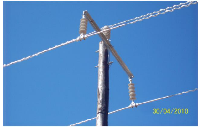
Figure 7: Another pole design, a single 22kV post insulator mounted on the top of a wood pole with suspended insulators. The structure does not offer much in the way of potential nest sites.
