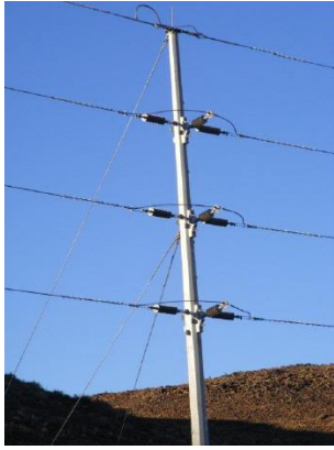
Figure 6: Detail at the top of the transmission pole showing minimal purchase for crow nests, but nevertheless nests are likely to be built.
