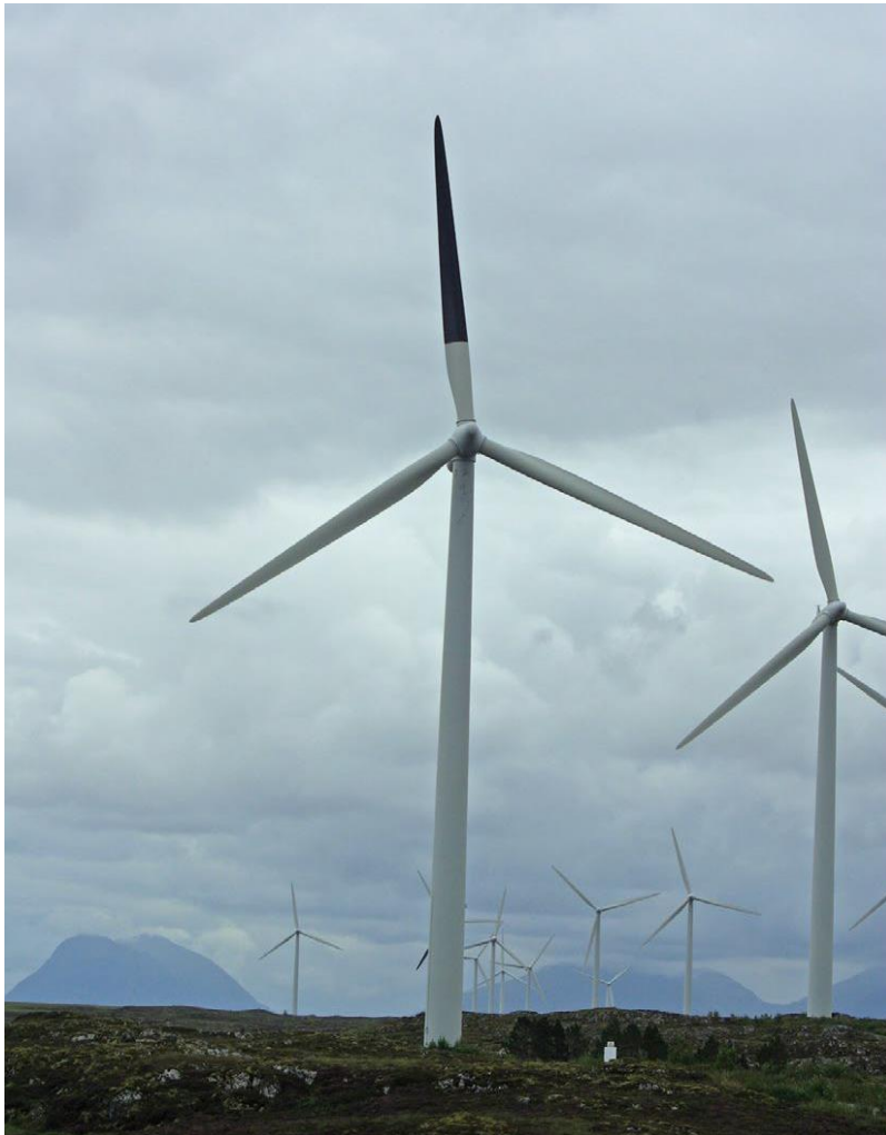
Figure 2: Turbine with painted blade in Norway (May et al. 2020)
