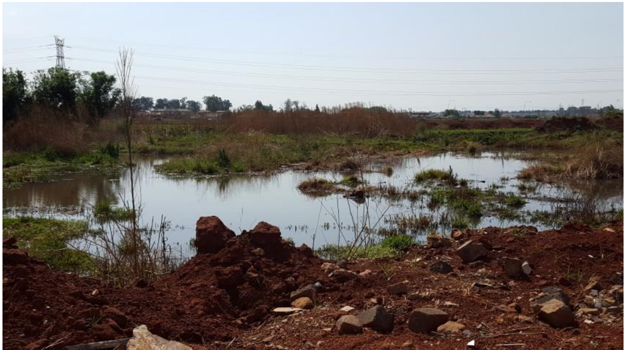
FIGURE 5: Accumulated water in the wetland area in the vicinity of the Trade Route substation
