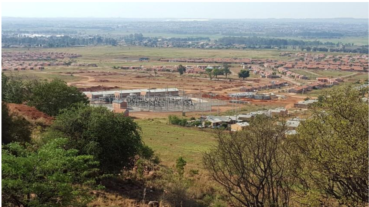
FIGURE 12: The Lehae substation and surrounding residential area
