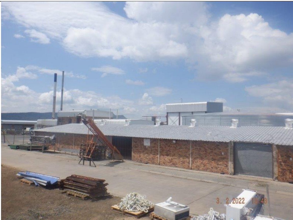
Figure 10: View of facility from scrapyard photograph 2
