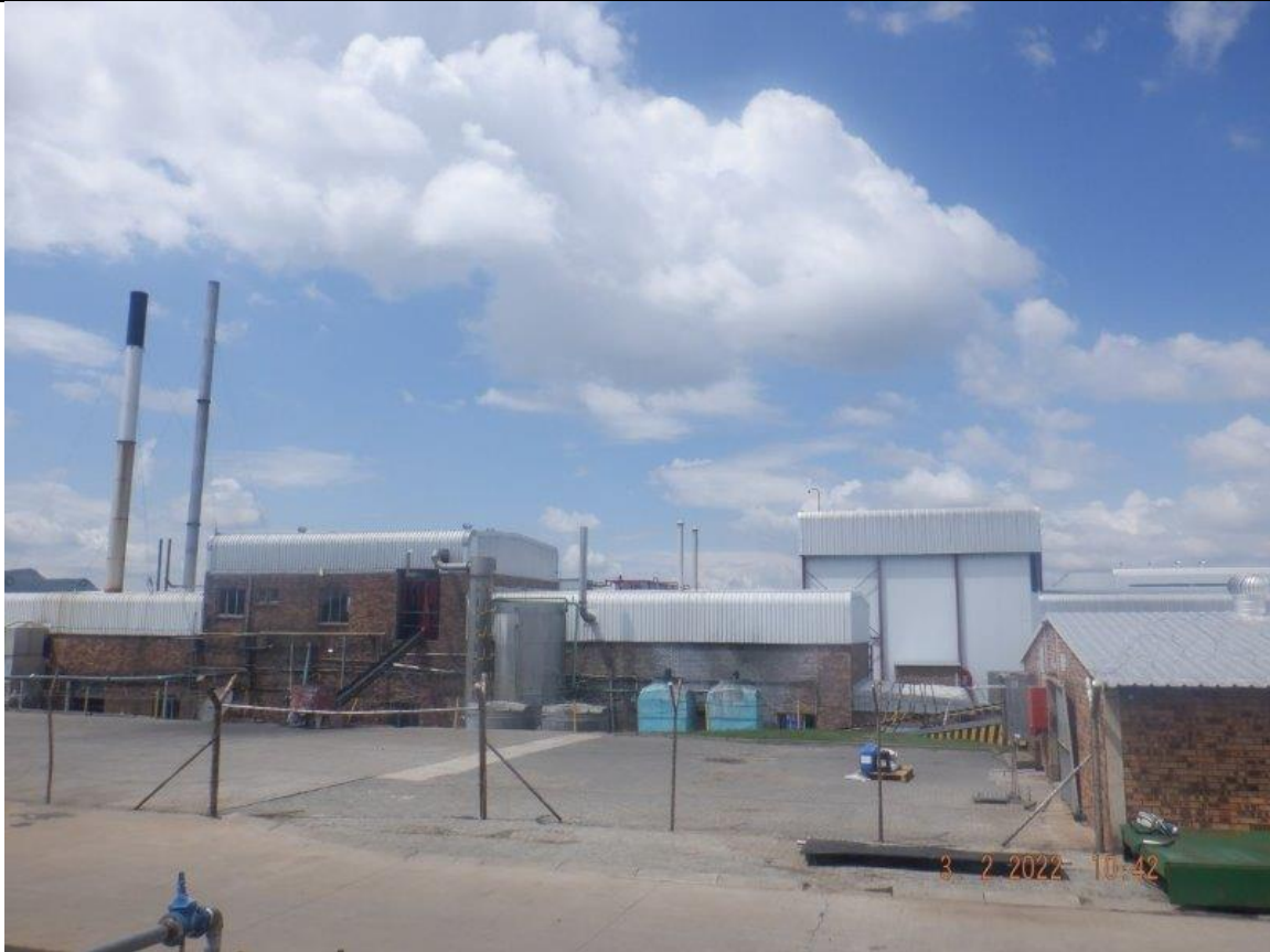
Figure 9: View of facility from scrapyard photograph 1
