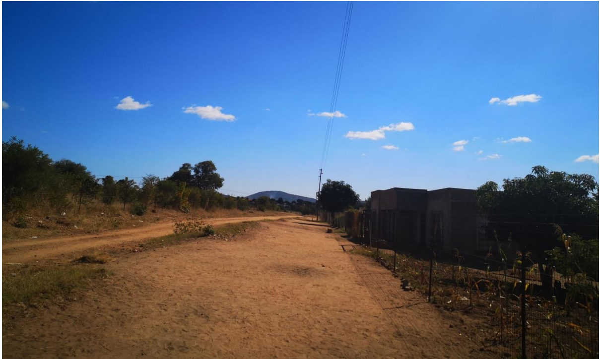
Existing powerline where the proposed will be connected
