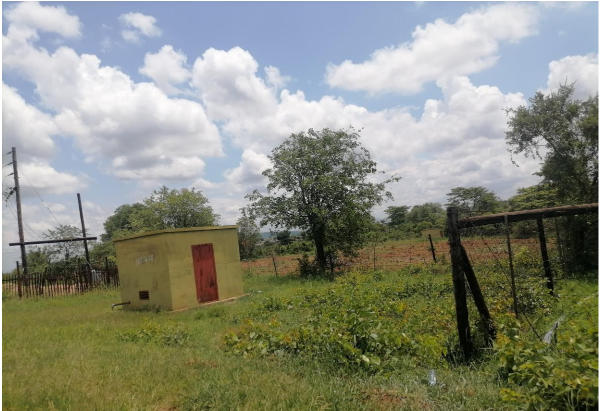
Photo 5: Shows the borehole where electricity will be connected
