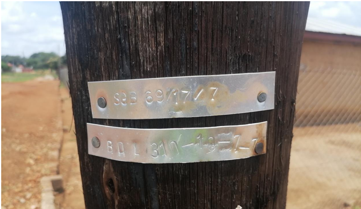
Photo 1: Shows the existing pole number on site
