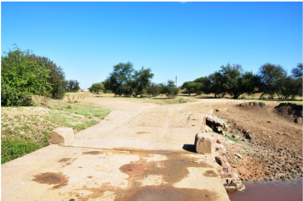
Bridge across Moretele river.
