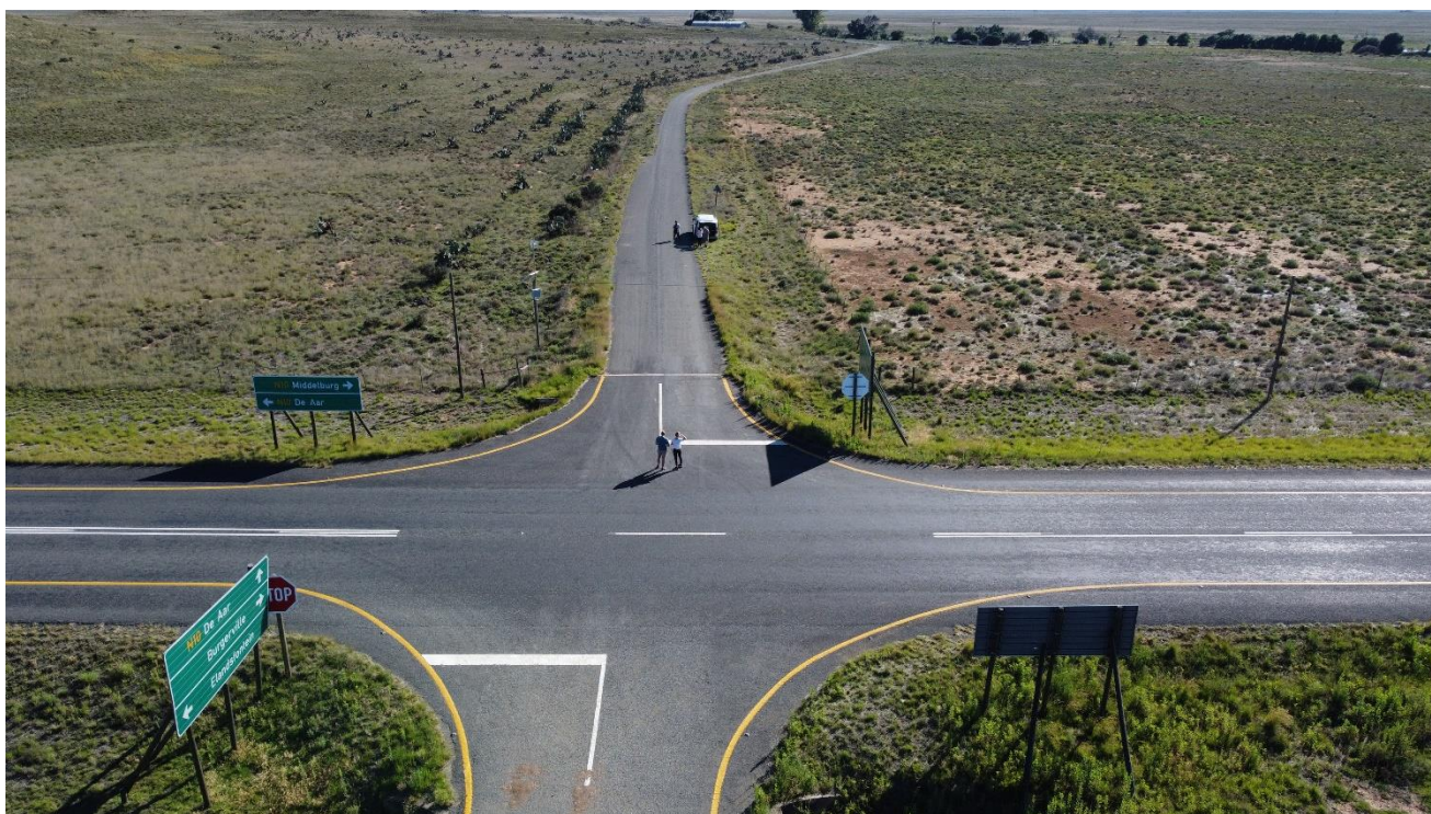
Photo 1: Start of the access road – N10/Burgerville public district road intersection (facing Northeast).
