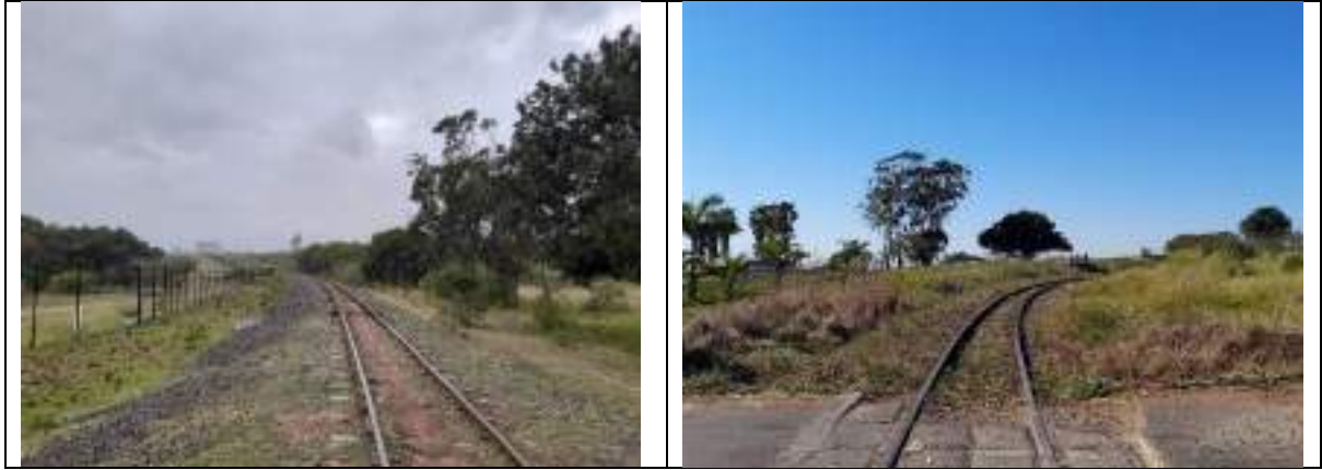
Railway track intersecting project area
