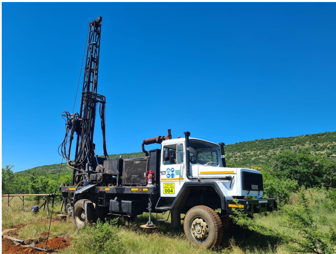
Photo Plate 3: Example of drill rig
