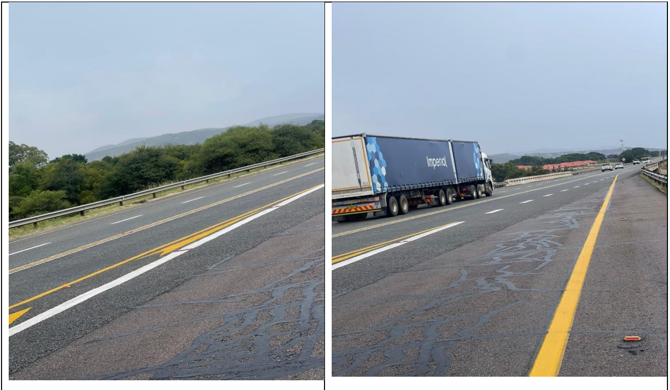
Photo 1: N4 National on portion 224 and 225
