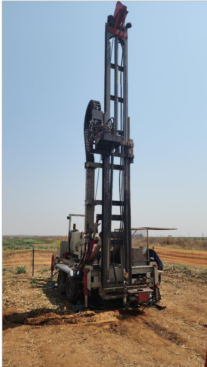
Figure 12: Example of drilling machinery.
