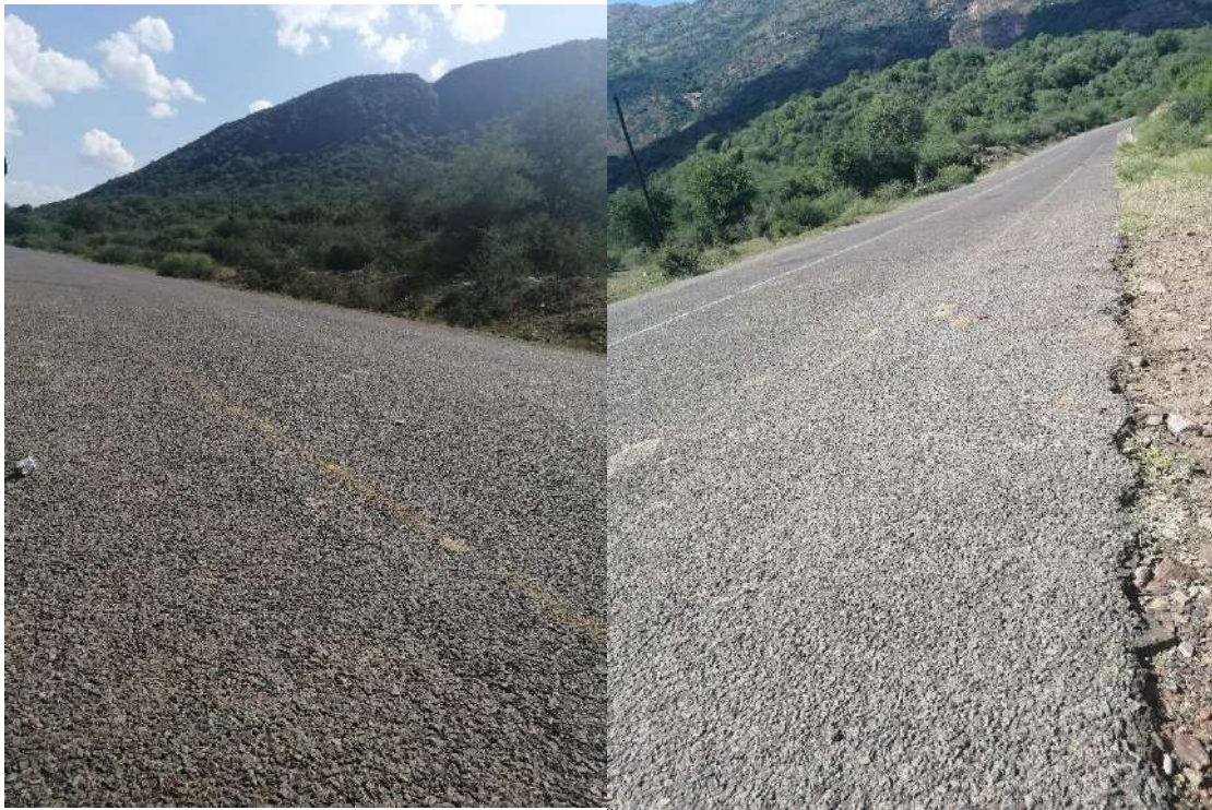
Figure 21: Sensitive receptor observed on site
