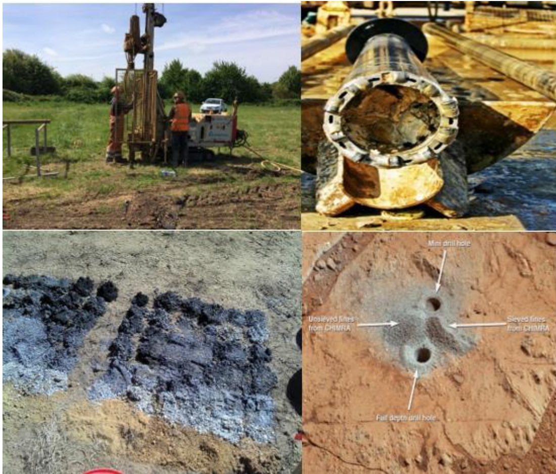
Figure 5: Typical example of drilling equipment and site setting
