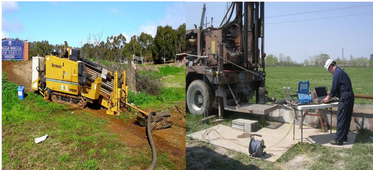
Figure 8: Directional drilling and Geophysical down-hole survey
