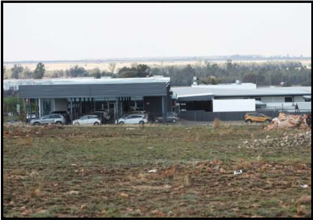
Photo 3 View of part of the site and built-up areas beyond the site. Photo: R.F. Terblanche.
