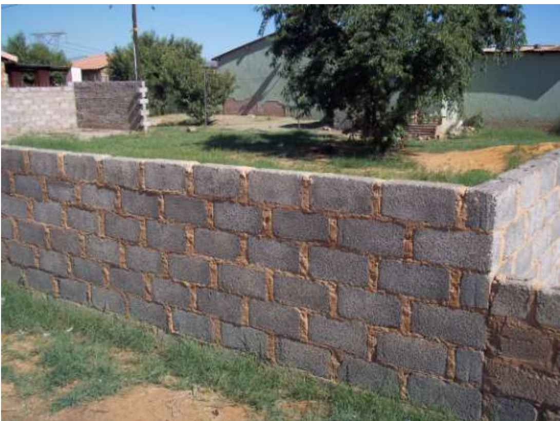
Photo 4: South-eastern perspective of the sewer connector line.
