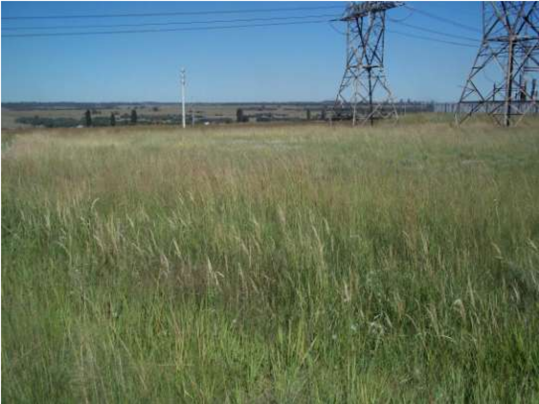
Photo 3: Eastern perspective of the sewer connector line.
