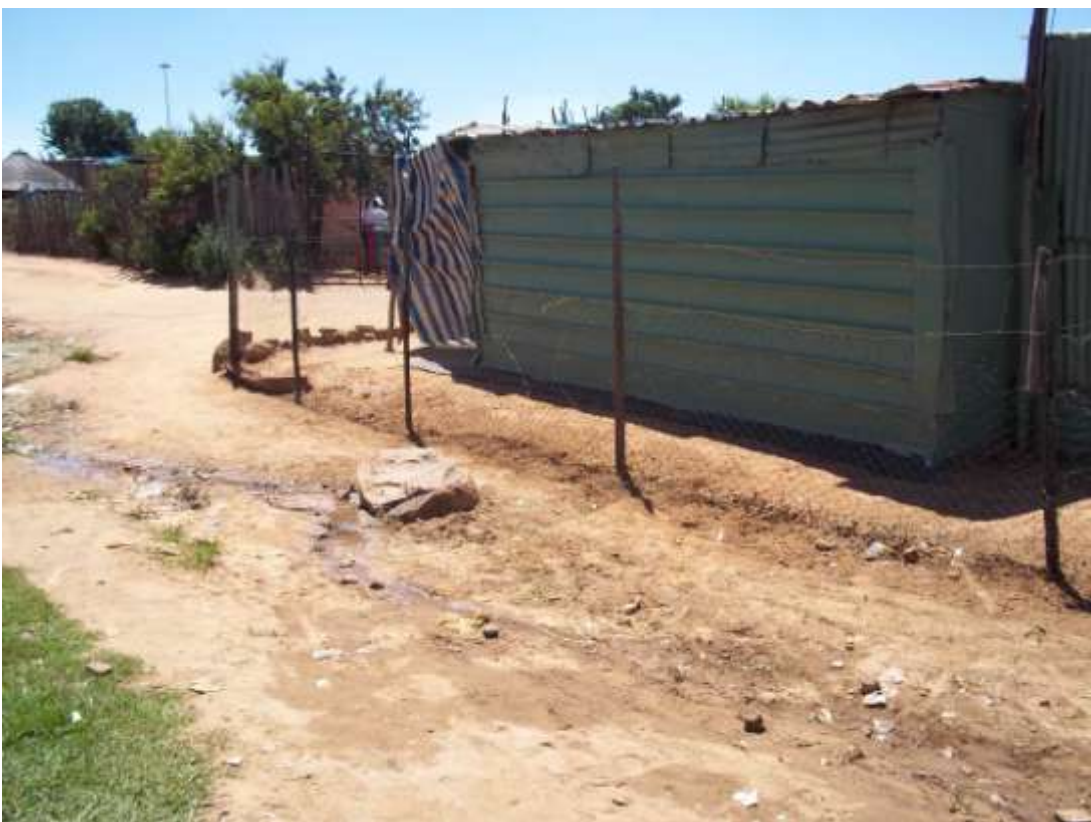
Photo 8: North-western perspective of the sewer connector line.
