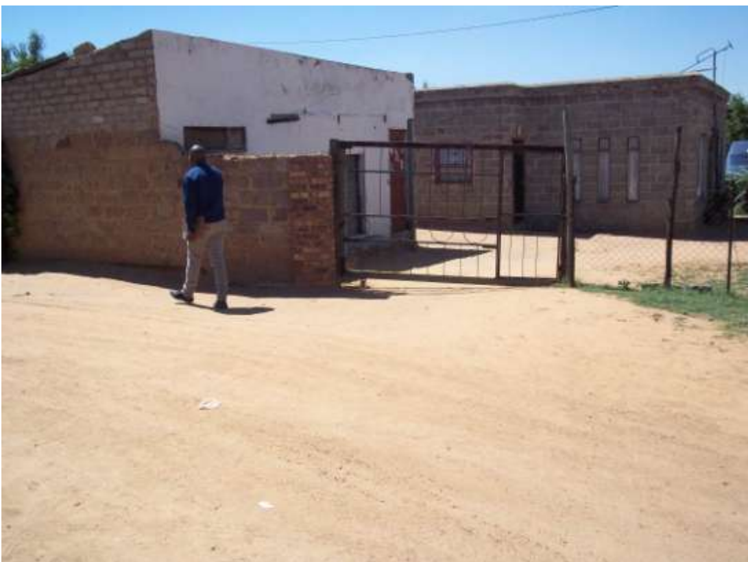
Photo 8: North-western perspective of the sewer connector line.
