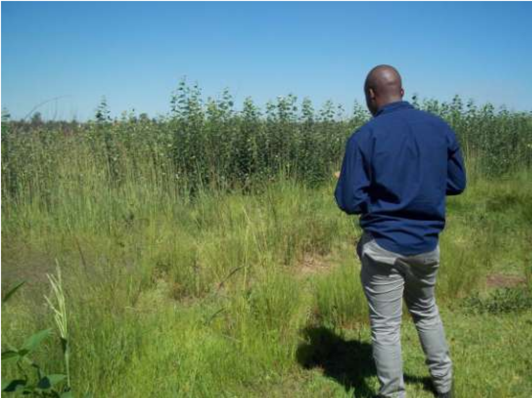
Photo 3: Eastern perspective of the sewer connector line.
