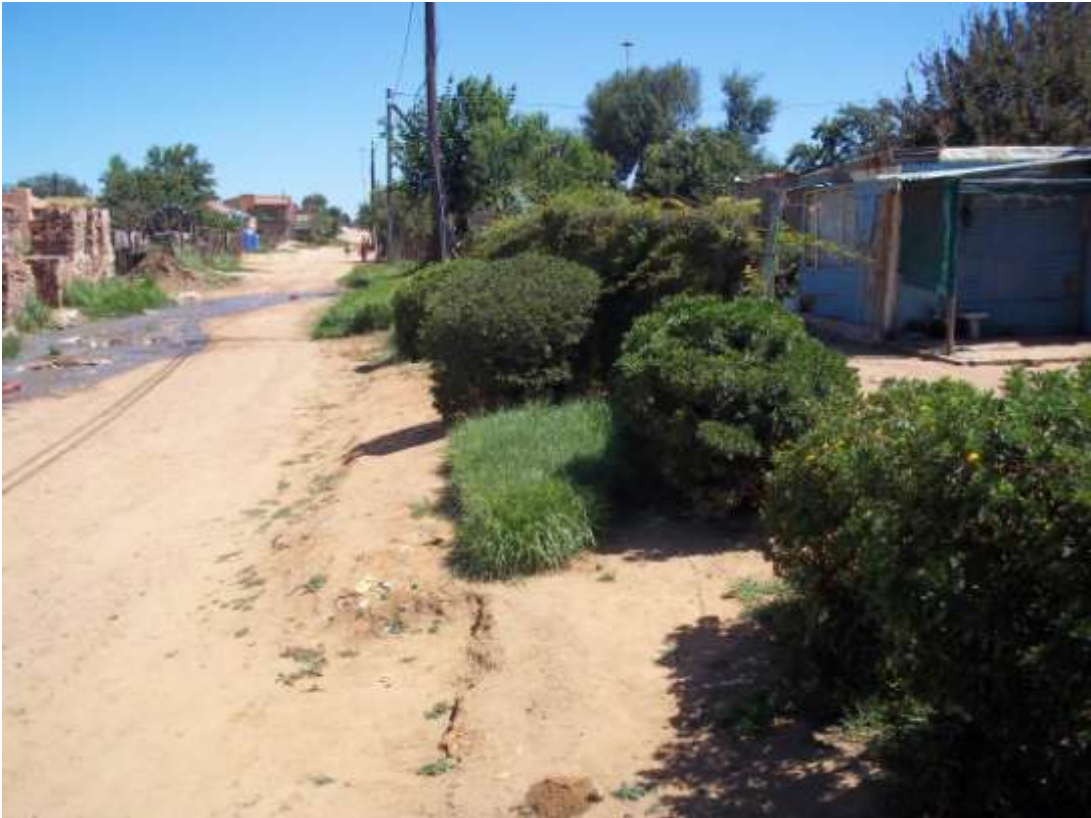
Photo 5: Southern perspective of the sewer connector line.
