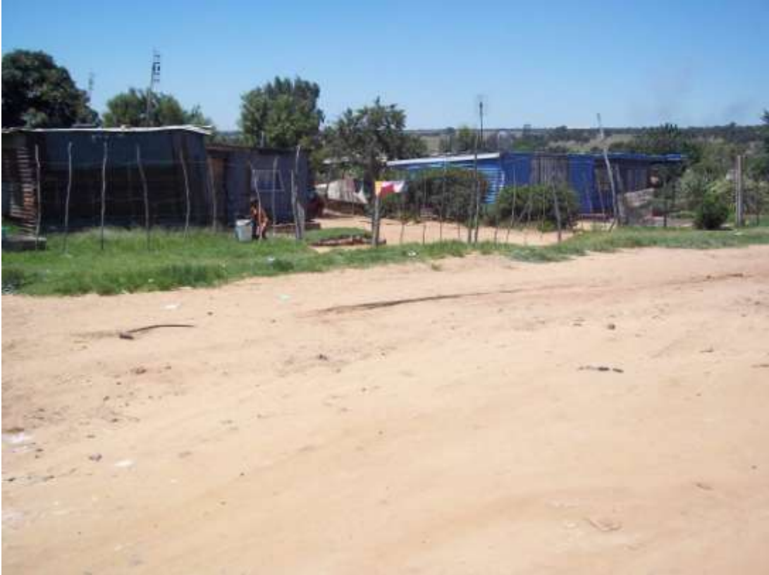
Photo 1: Northern perspective of the sewer connector line.
