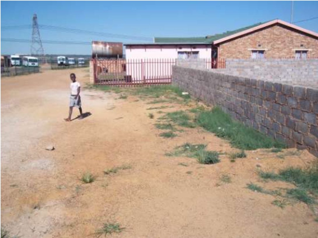
Photo 3: Eastern perspective of the sewer connector line.
