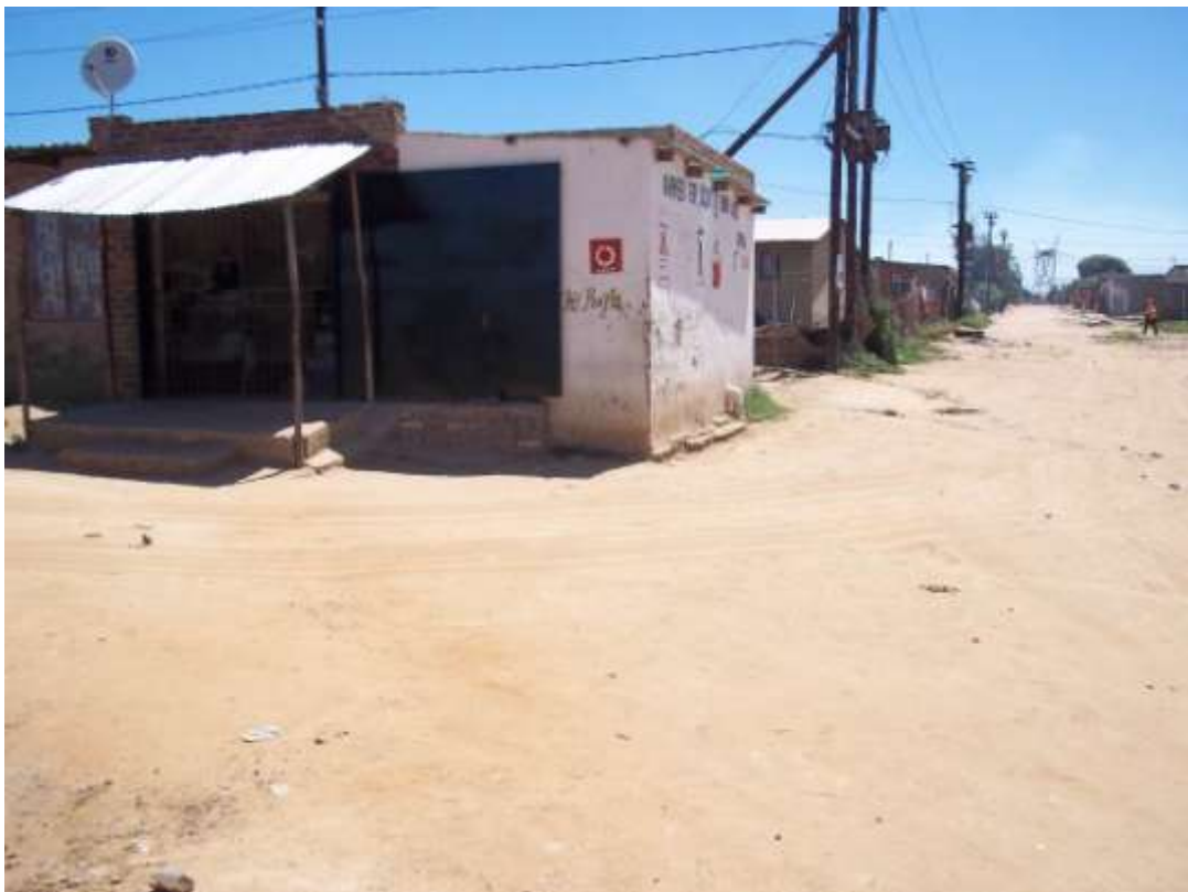
Photo 6: South-western perspective of the sewer connector line.
