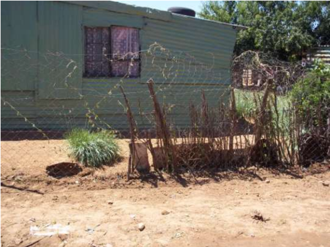
Photo 1: Northern perspective of the sewer connector line.
