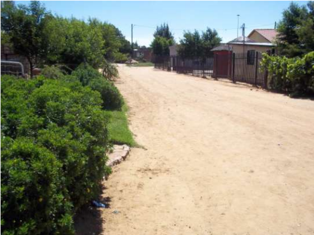
Photo 7: Western perspective of the sewer connector line.
