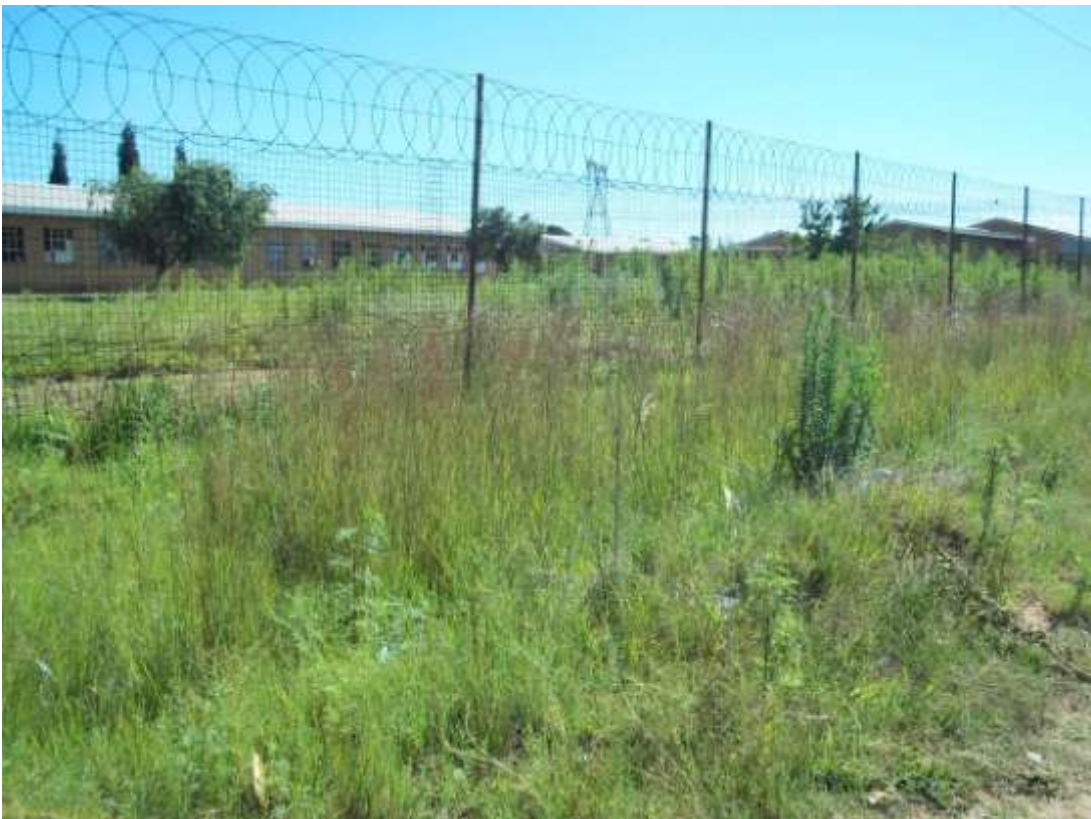
Photo 6: South-western perspective of the sewer connector line.
