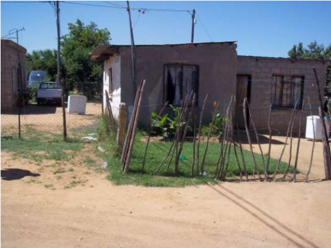
Photo 1: Northern perspective of the sewer connector line.
