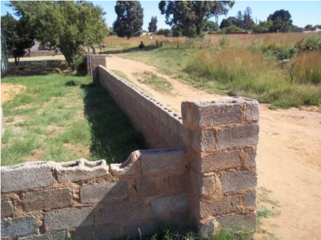
Photo 5: Southern perspective of the sewer connector line.
