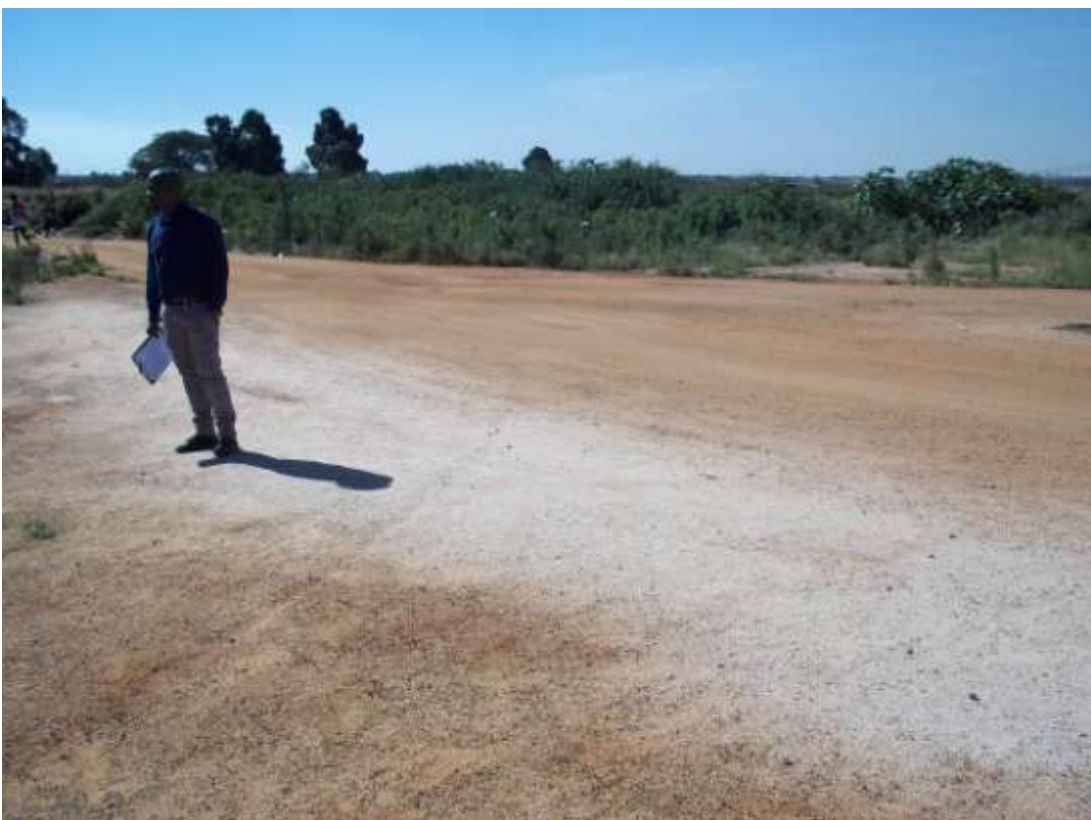
Photo 8: North-western perspective of the sewer connector line.
