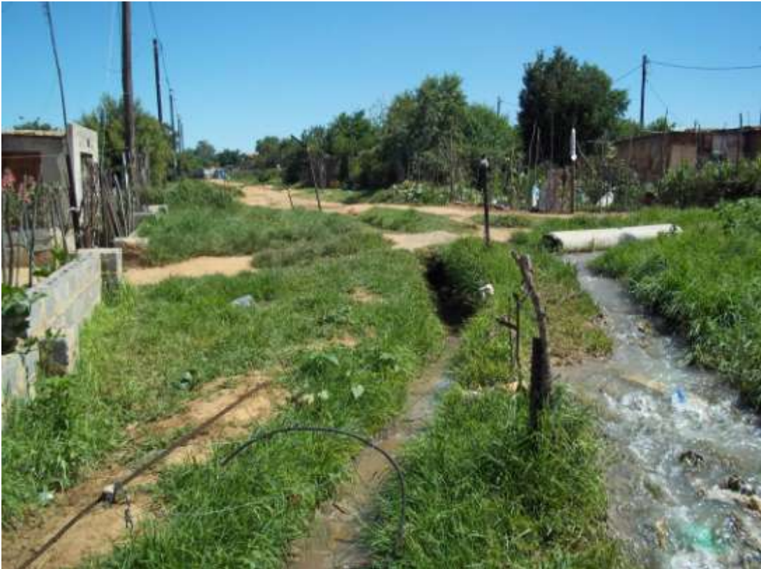
Photo 5: Southern perspective of the sewer connector line.
