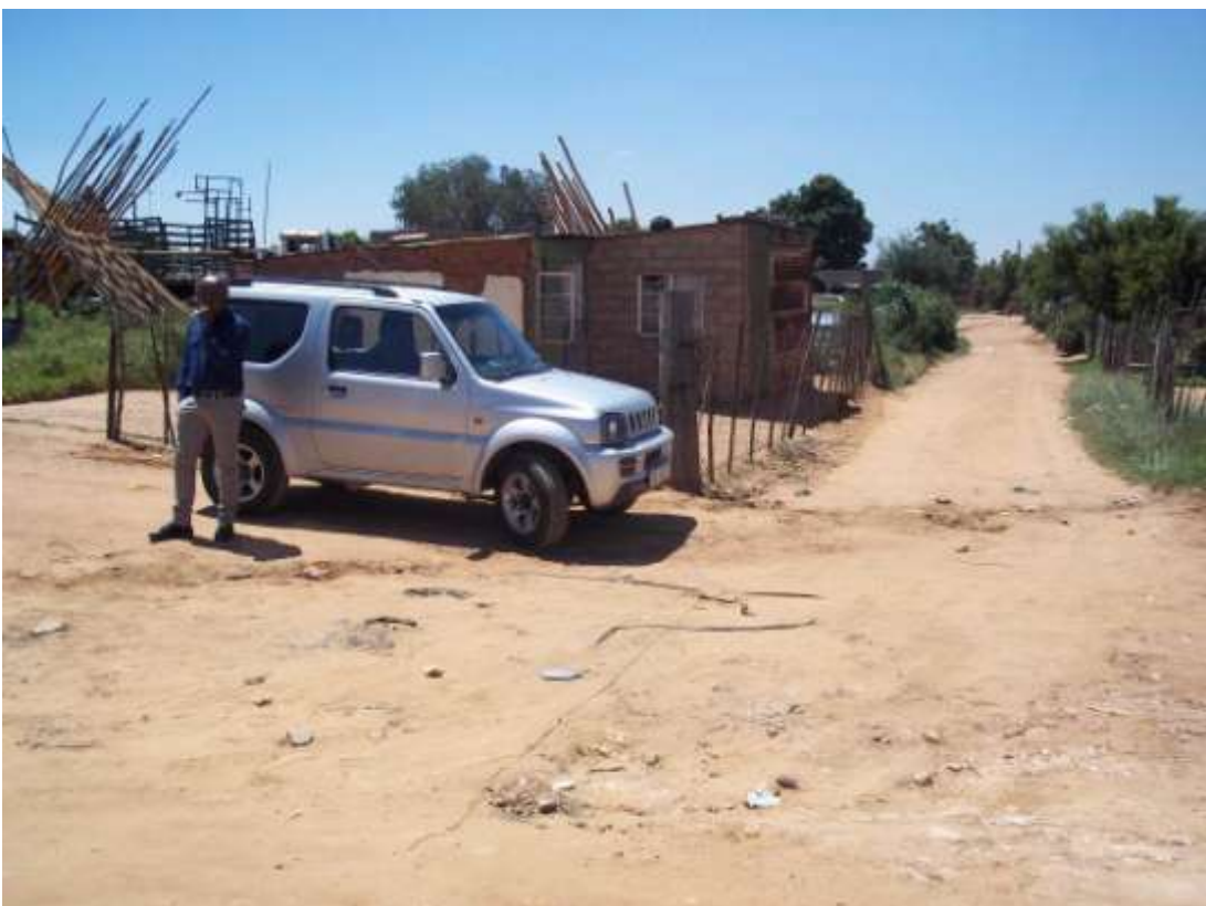
Photo 8: North-western perspective of the sewer connector line.
