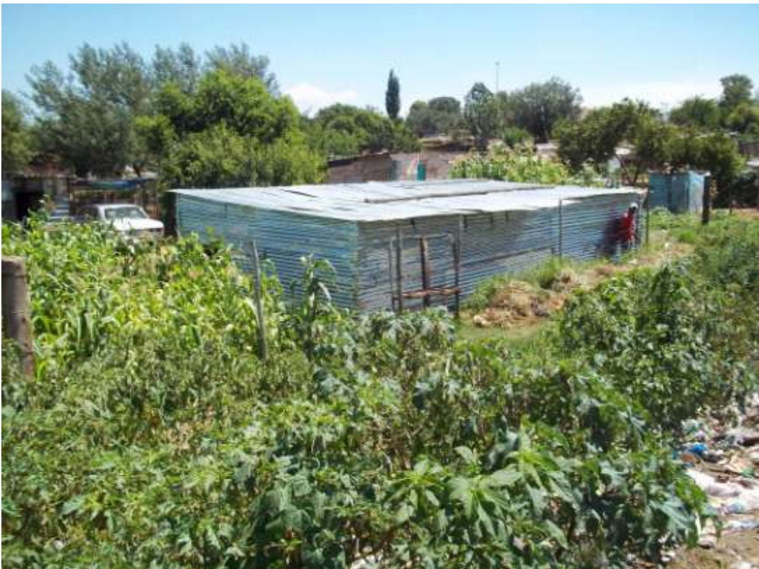
Photo 6: South-western perspective of the sewer connector line.
