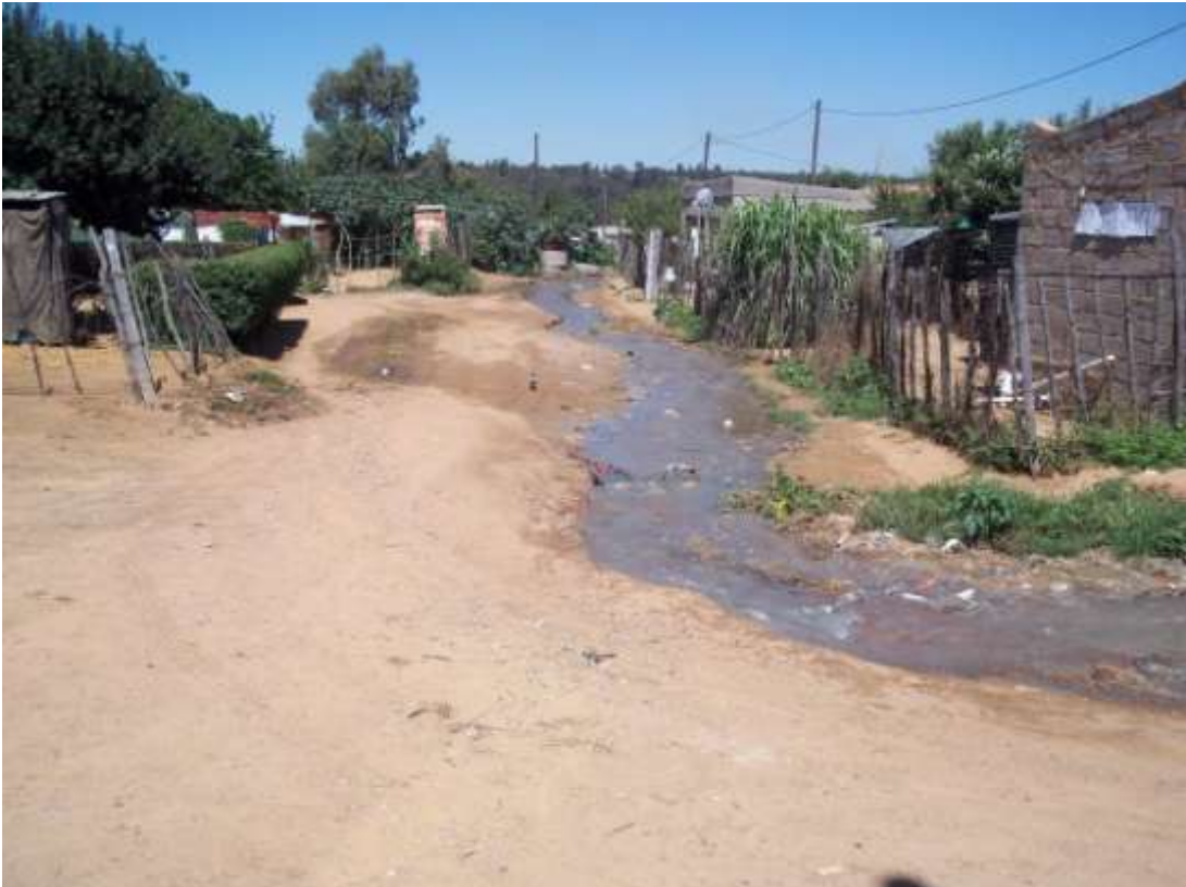
Photo 3: Eastern perspective of the sewer connector line.
