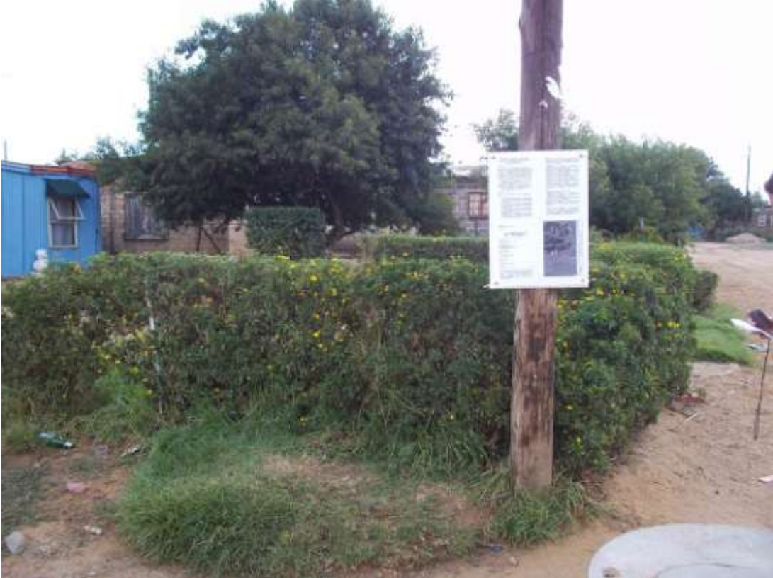
Photo 7: Location of the site notice on the street corner at the start of Sewer Collector Line No. 2.
