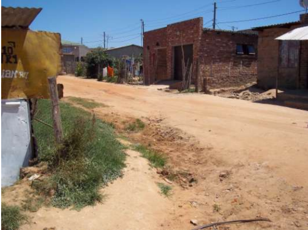
Photo 5: Southern perspective of the sewer connector line.
