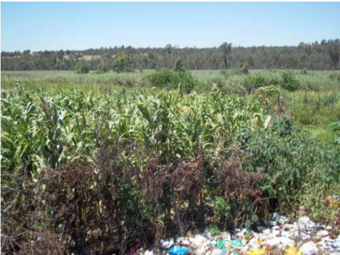
Photo 2: North-eastern perspective of the sewer connector line.
