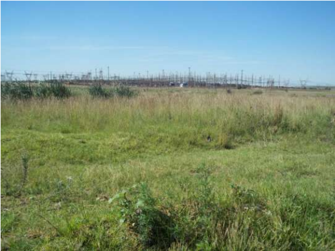
Photo 1: Northern perspective of the sewer connector line.
