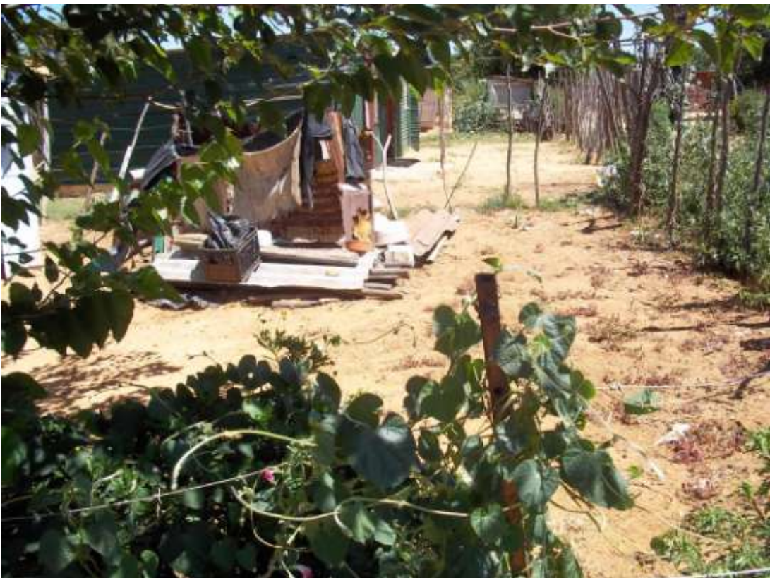
Photo 4: South-eastern perspective of the sewer connector line.
