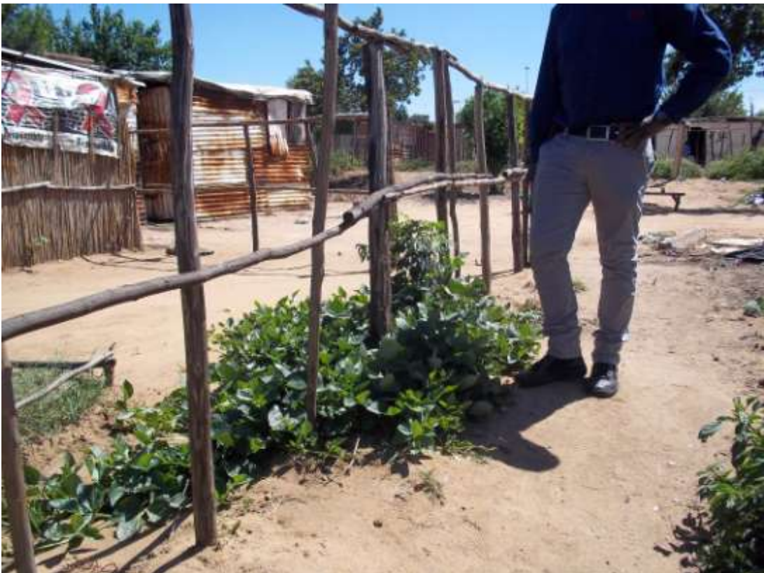
Photo 6: South-western perspective of the sewer connector line.
