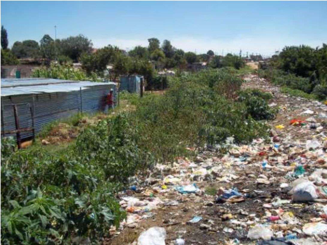
Photo 7: Western perspective of the sewer connector line.
