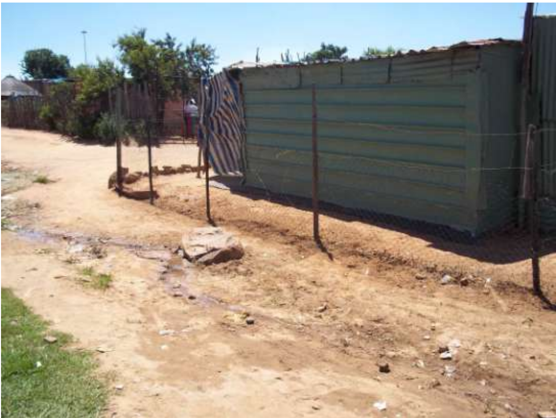
Photo 8: North-western perspective of the sewer connector line.
