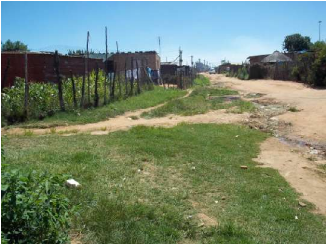
Photo 7: Western perspective of the sewer connector line.
