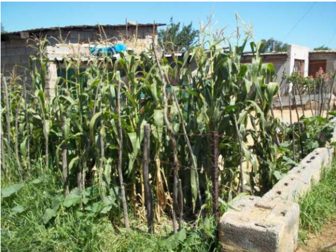
Photo 4: South-eastern perspective of the sewer connector line.
