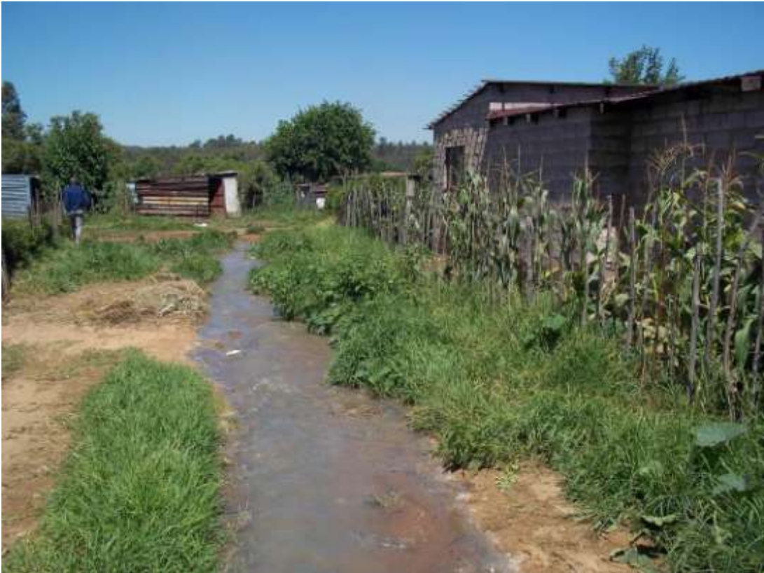
Photo 3: Eastern perspective of the sewer connector line.
