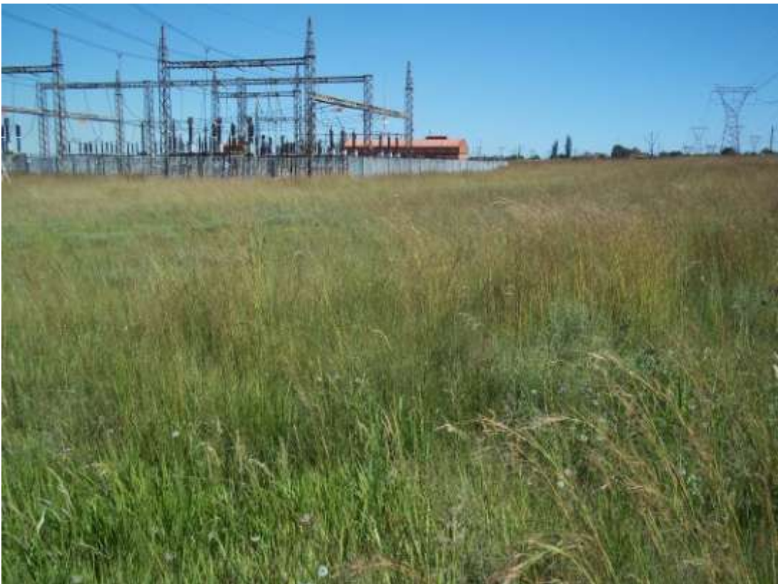
Photo 4: South-eastern perspective of the sewer connector line.
