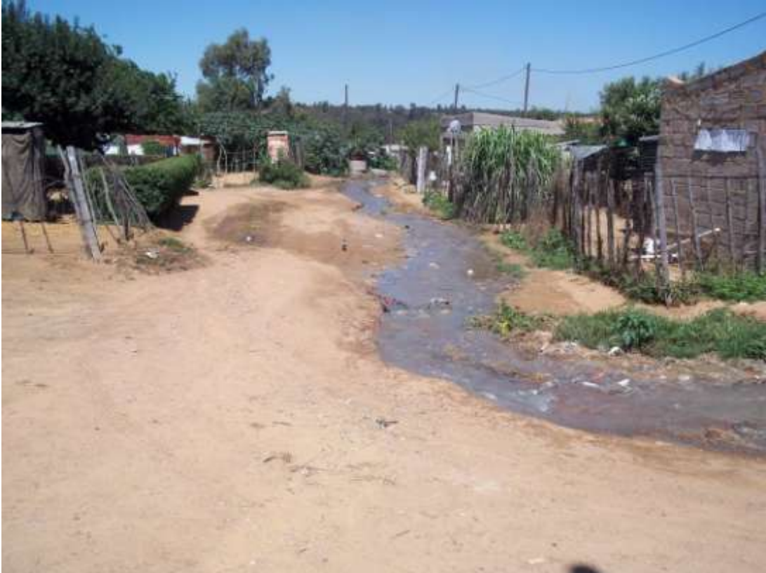
Photo 3: Eastern perspective of the sewer connector line.
