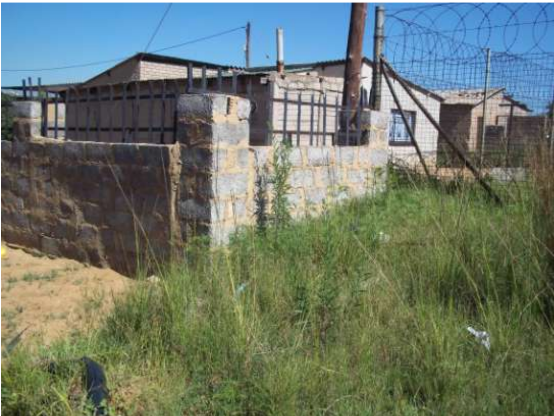
Photo 4: South-eastern perspective of the sewer connector line.
