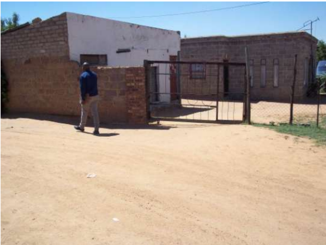
Photo 8: North-western perspective of the sewer connector line.
