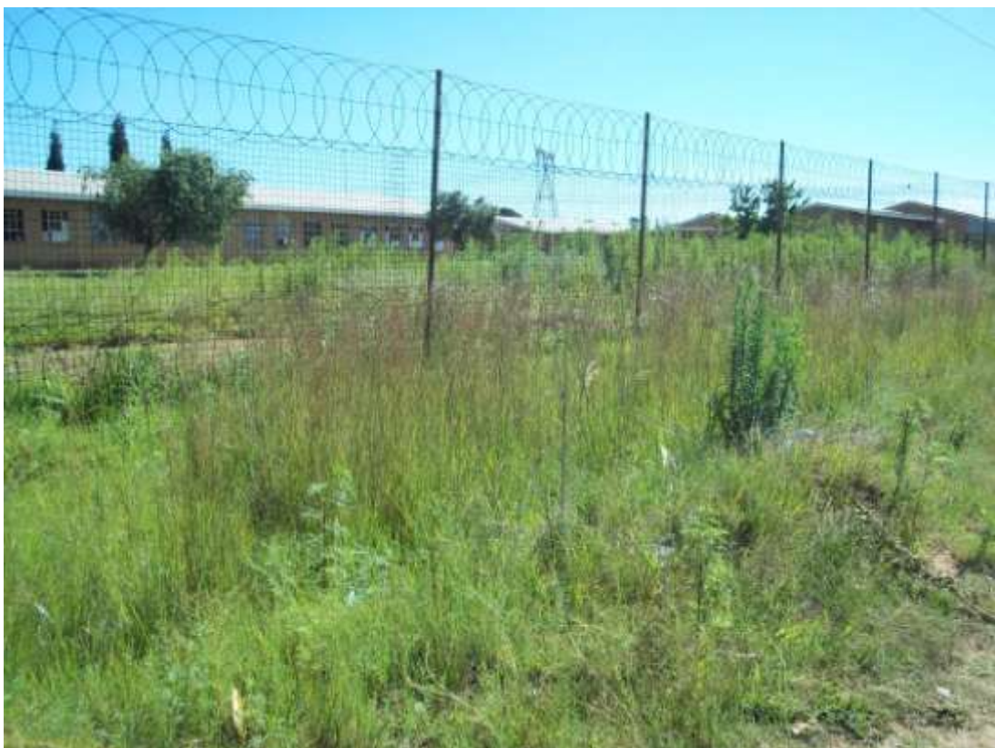
Photo 6: South-western perspective of the sewer connector line.
