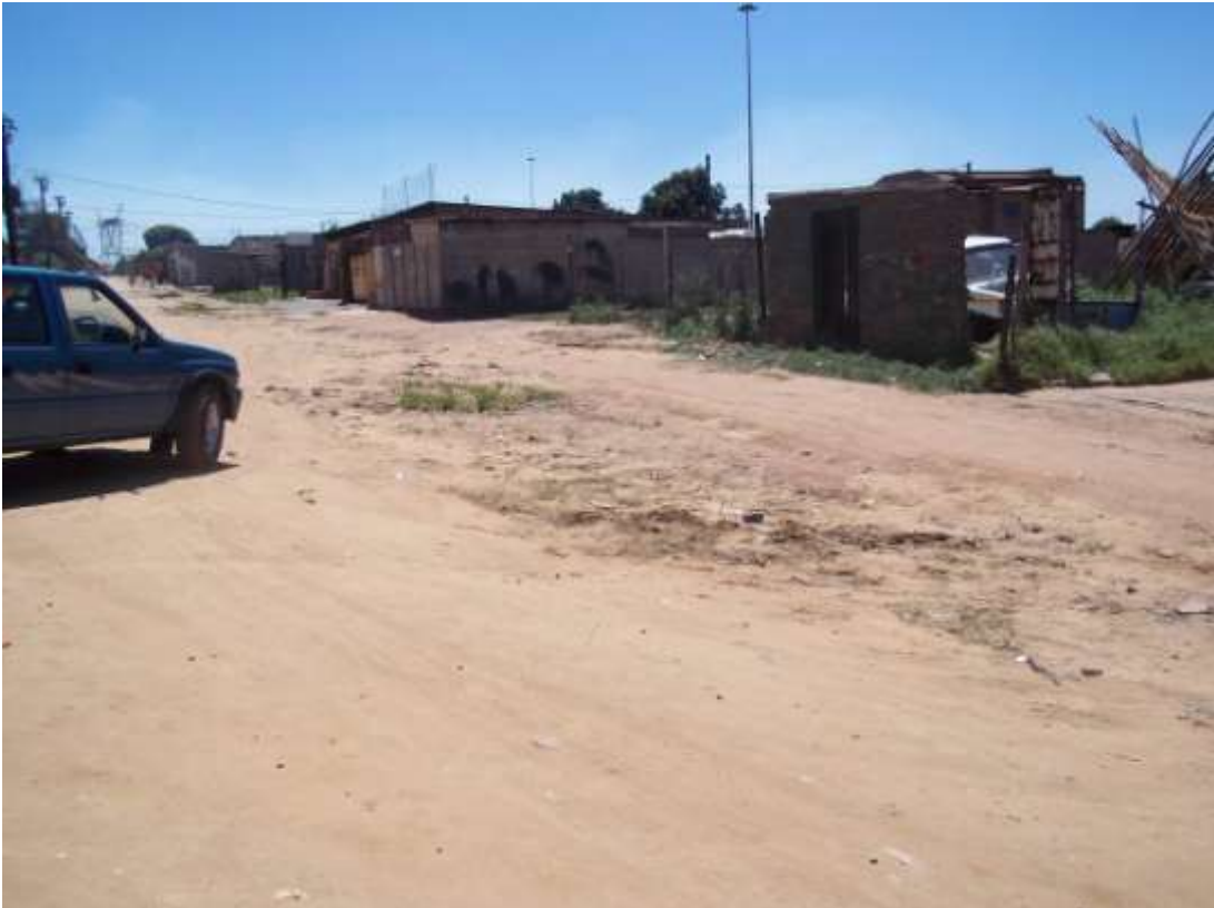
Photo 7: Western perspective of the sewer connector line.
