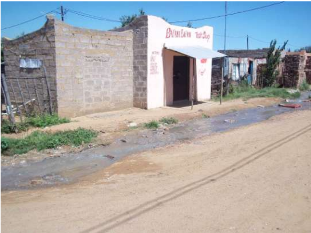
Photo 4: South-eastern perspective of the sewer connector line.
