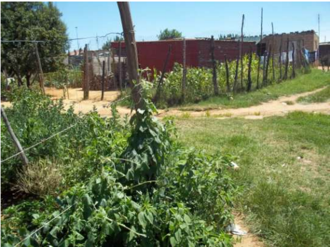
Photo 6: South-western perspective of the sewer connector line.
