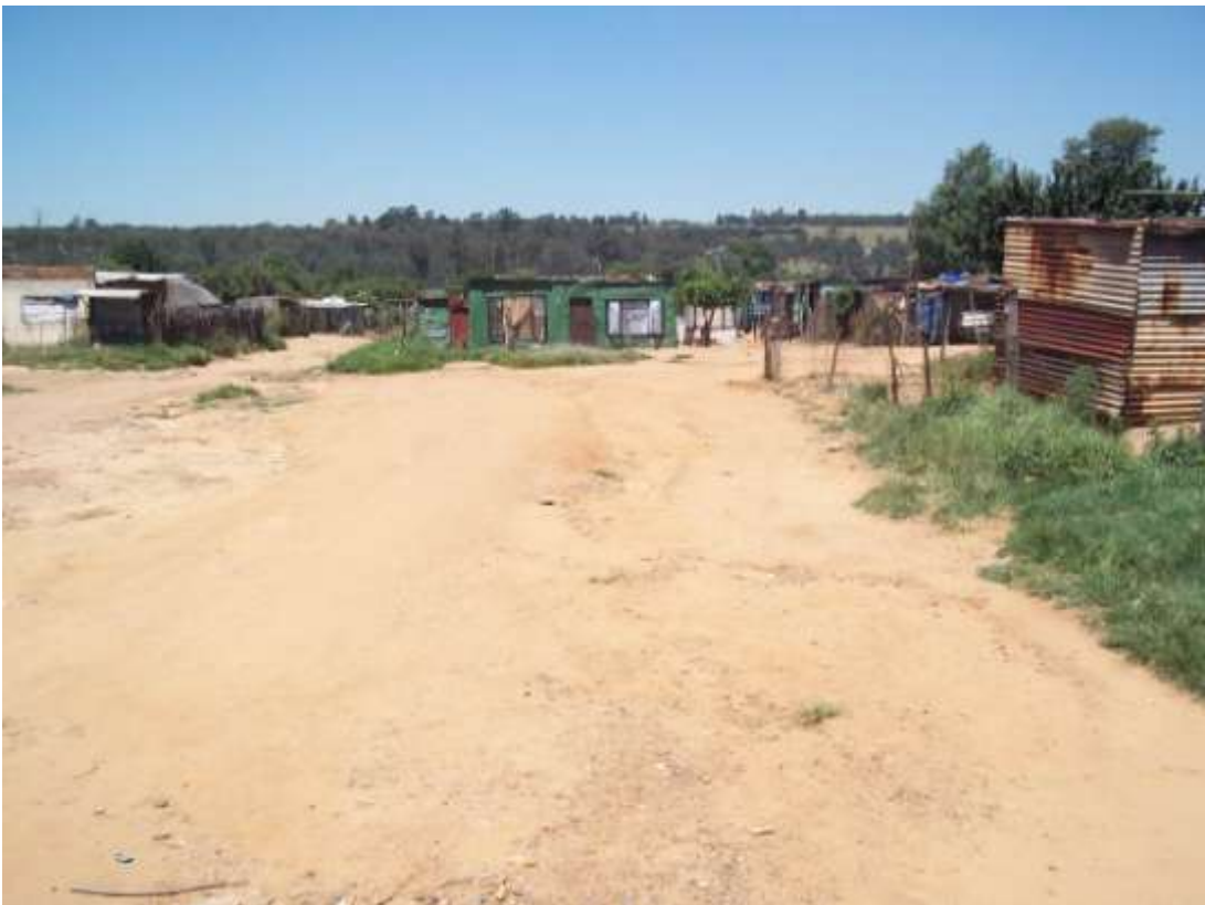
Photo 2: North-eastern perspective of the sewer connector line.
