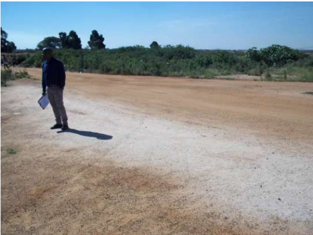
Photo 8: North-western perspective of the sewer connector line.
