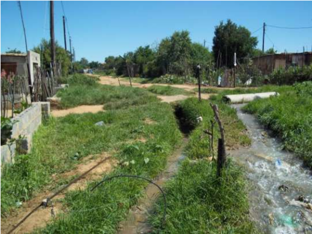
Photo 5: Southern perspective of the sewer connector line.
