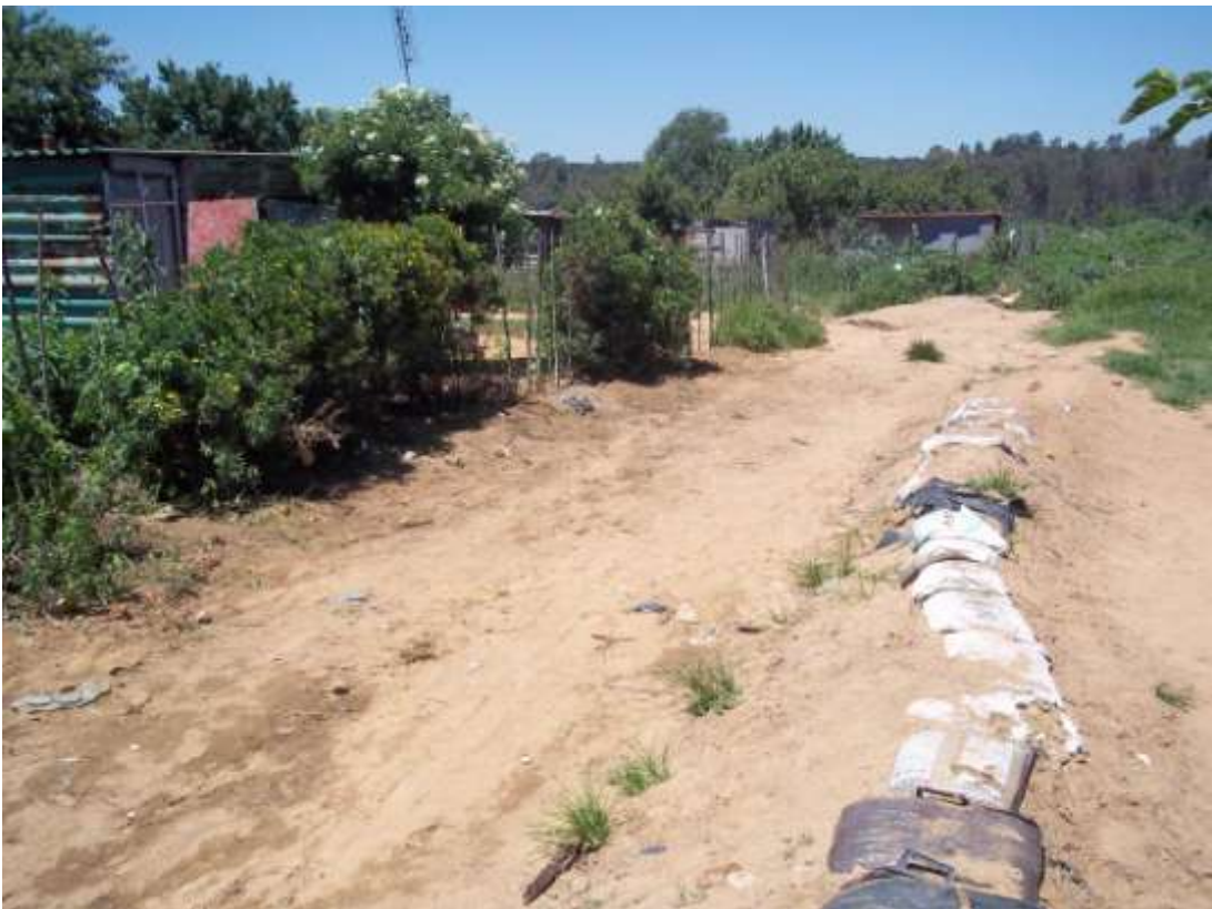
Photo 2: North-eastern perspective of the sewer connector line.
