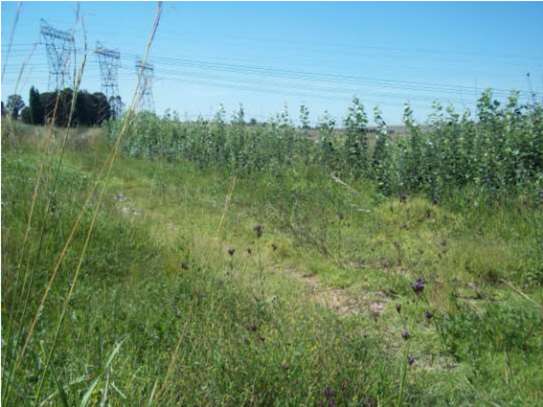
Photo 1: Northern perspective of the sewer connector line.
