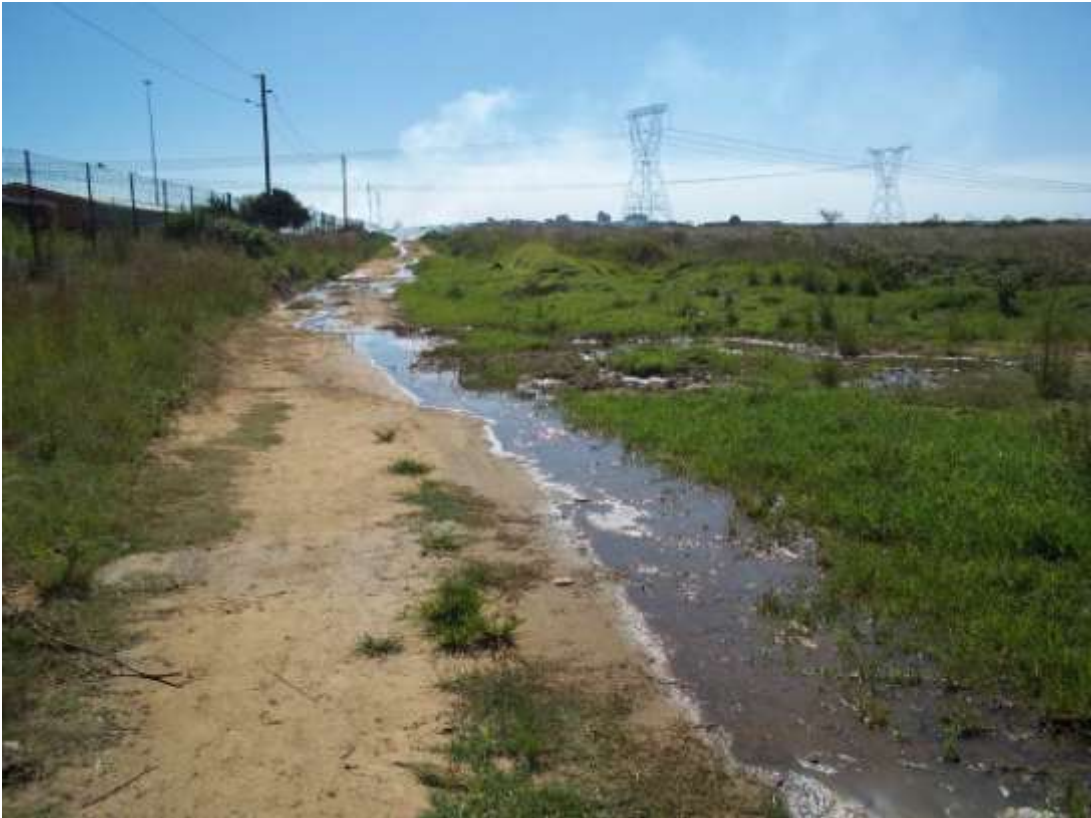
Photo 7: Western perspective of the sewer connector line.
