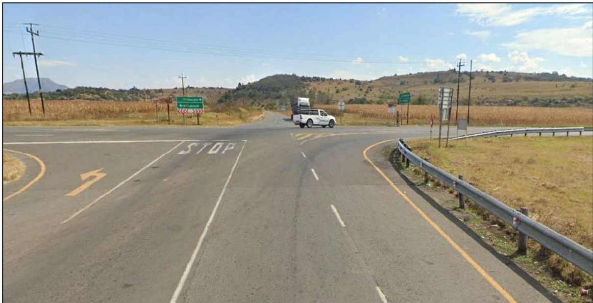
Figure 3-4: The R621 and N11 junction at the site
