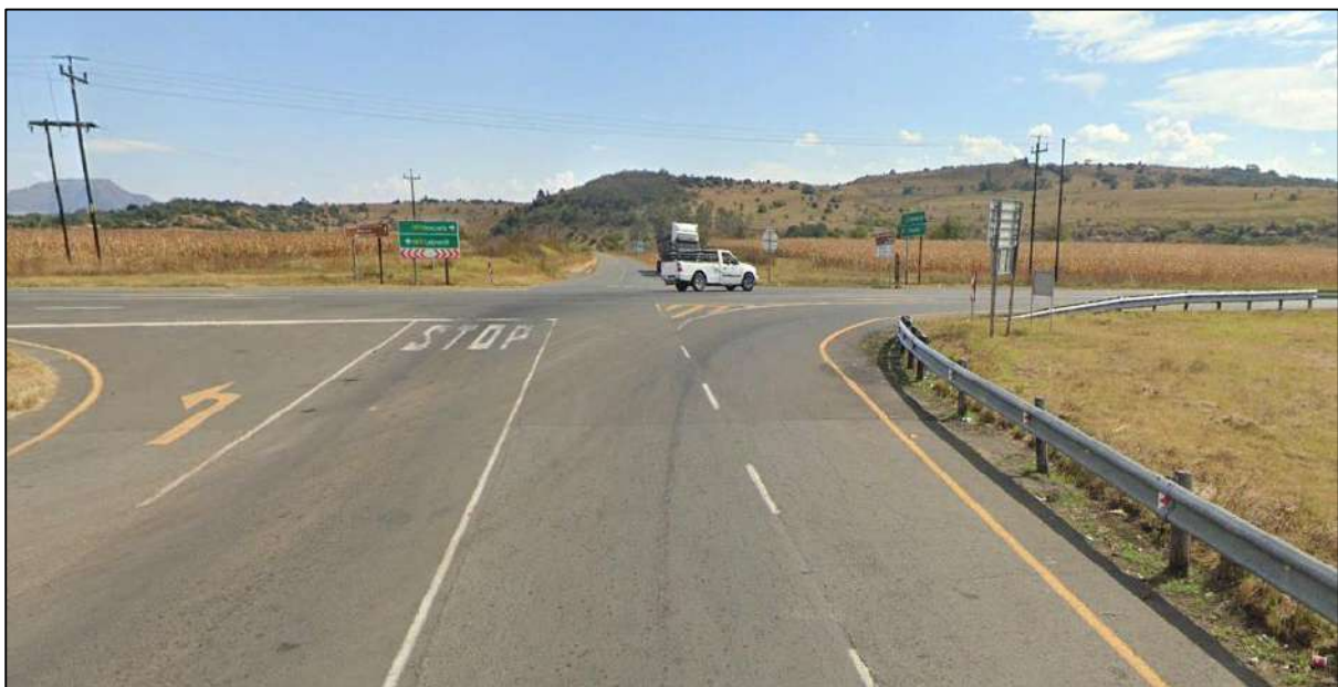
Figure 2-4: The R621 and N11 junction at the site
