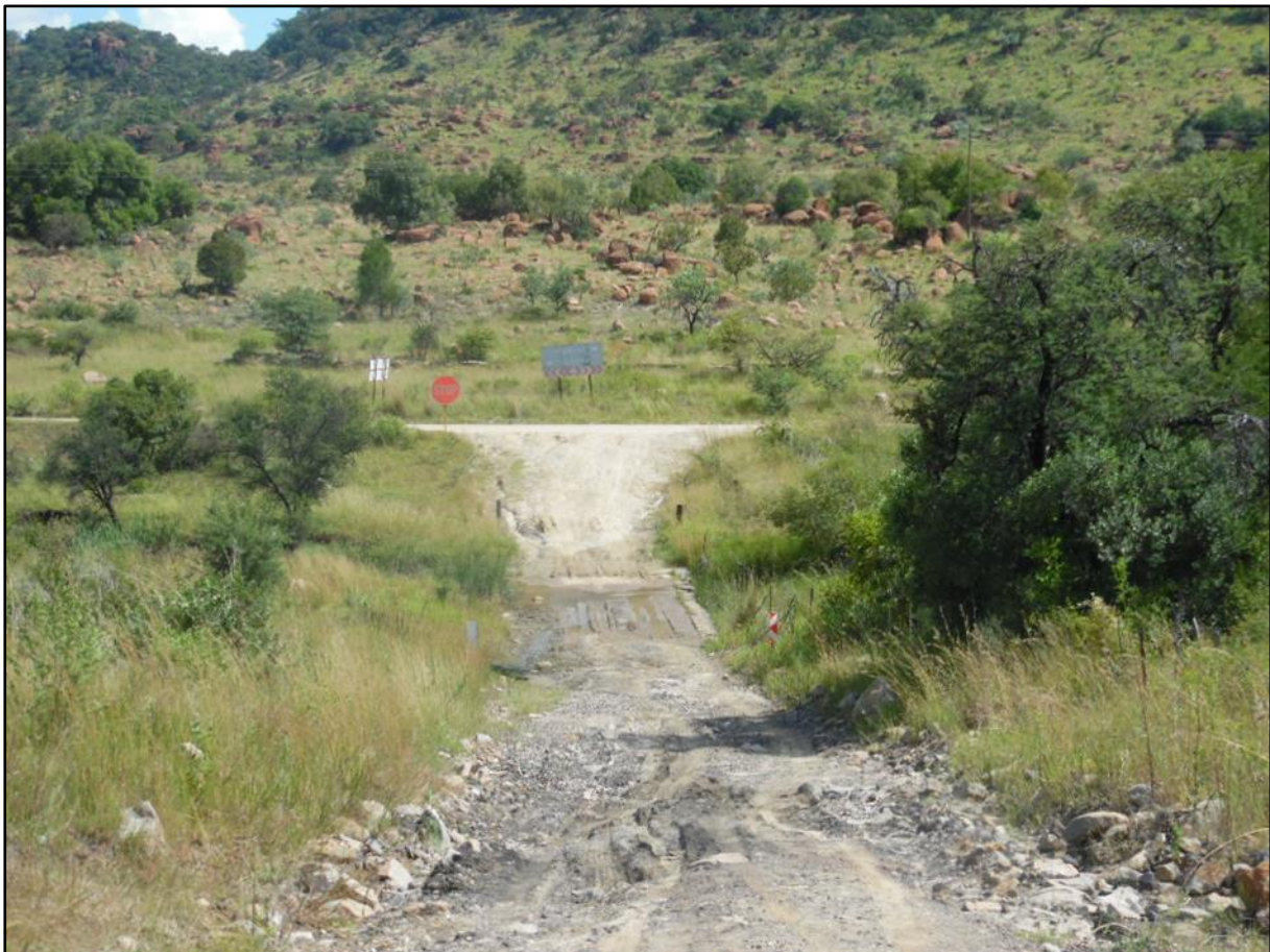
Figure 3-3: View of the site gravel access road
