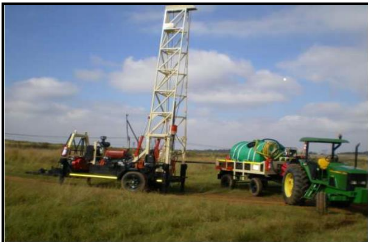
Figure 1-3: Typical LY44 Geological core drill unit
