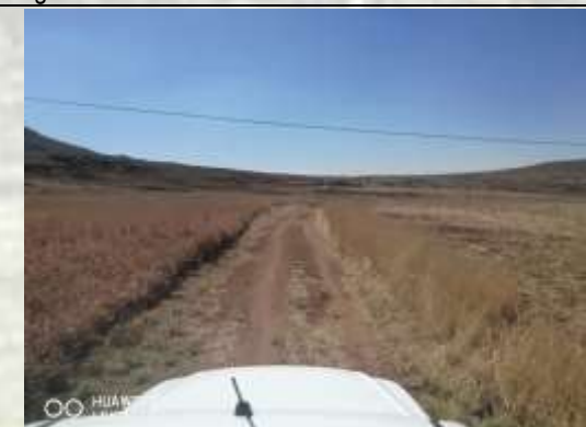
Figure 4: Mbilane access road towards the end.
