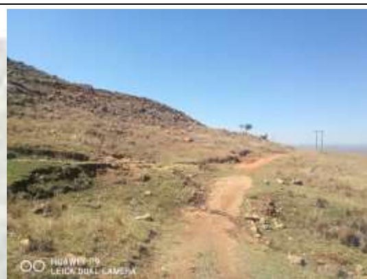
Figure 2: Mbilane access road mid section.
