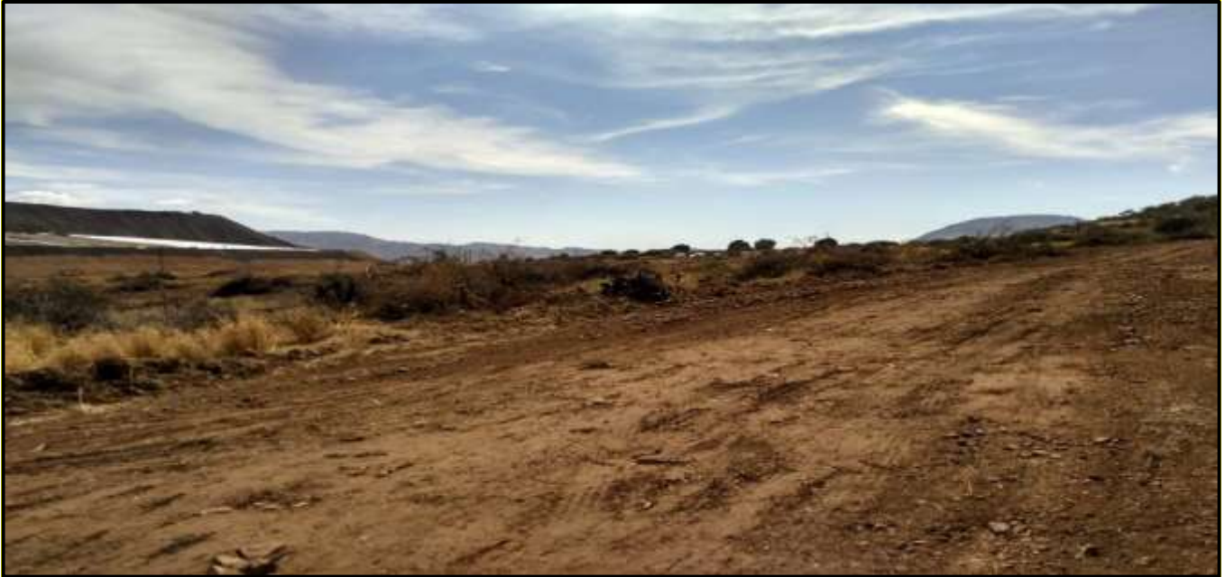
Figure 8: View towards the north-west, newly created access roads are visible
