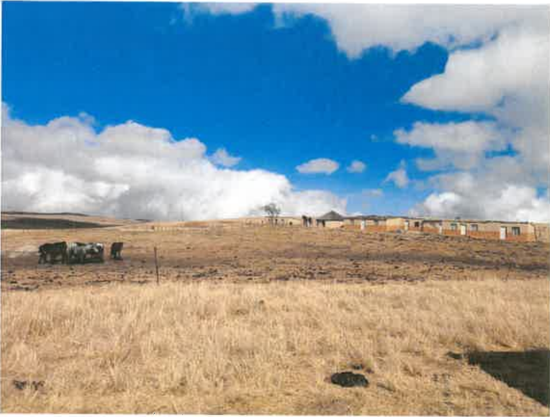
Photo 6.3-1: An example of the families' current houses
