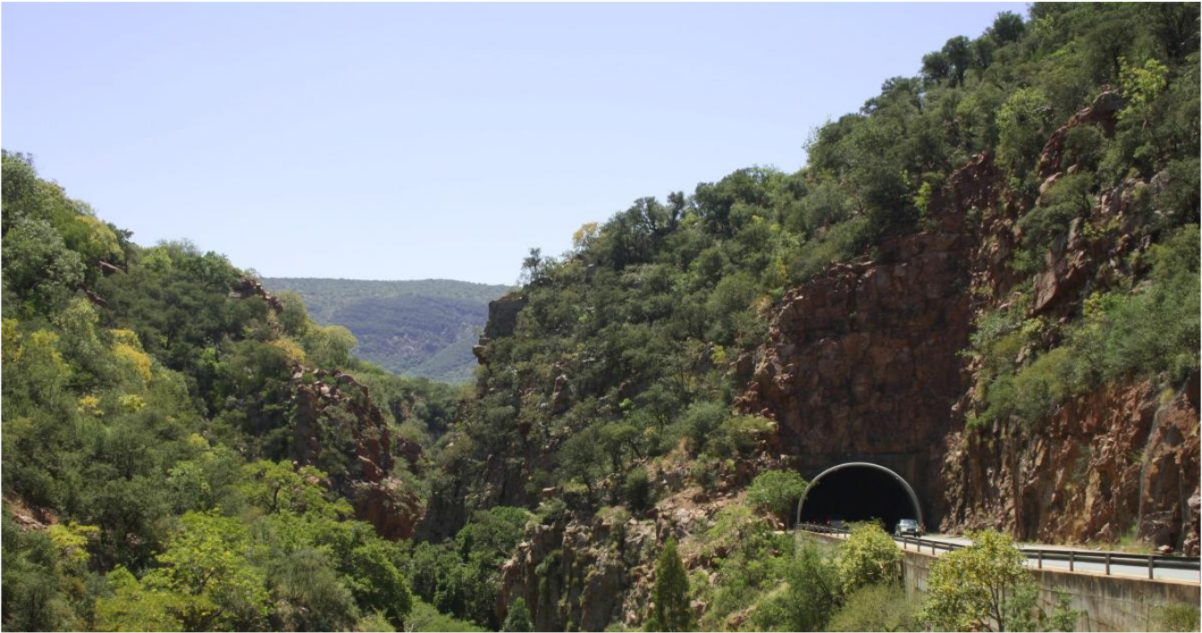
Figure 1.1 Cliffs and valleys of the Soutpansberg, with the Hendrik Verwoerd tunnel.
