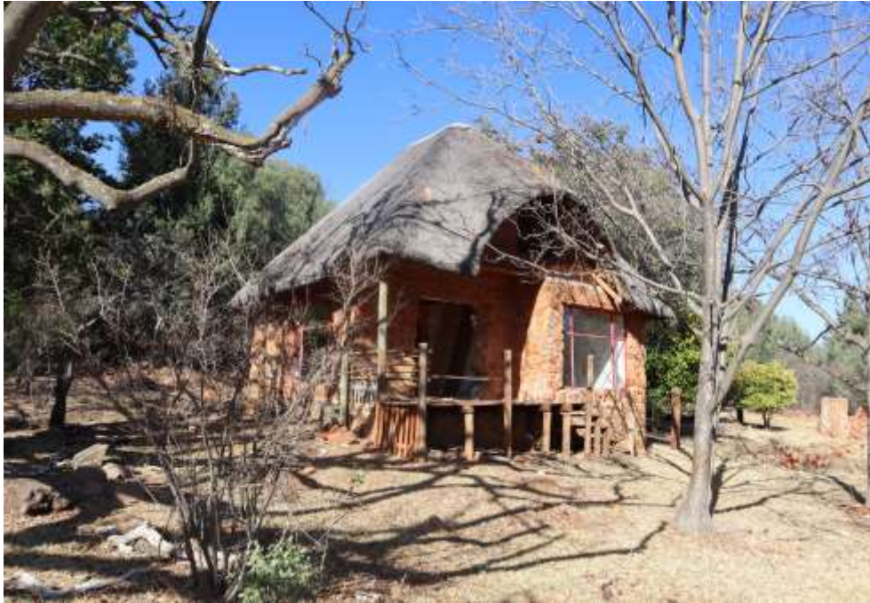
Figure 21: Vandalized thatched house.
