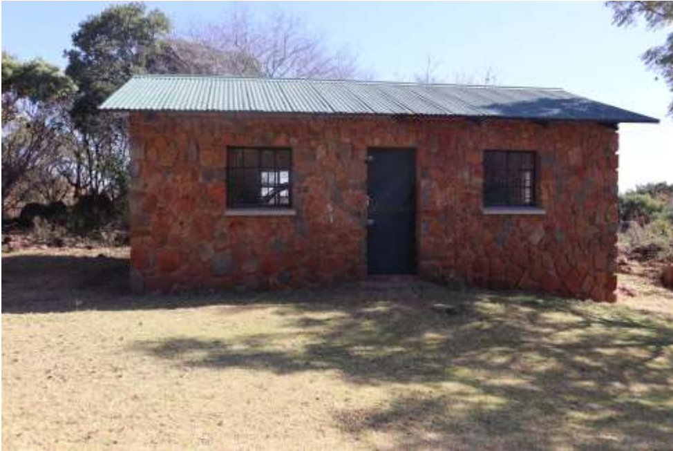
Figure 25: View of the farm laborer camp.
