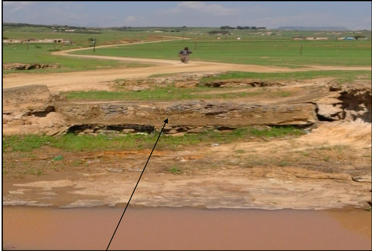
Photo 4: Showing existing gabion structure for erosion control along the stream banks.
