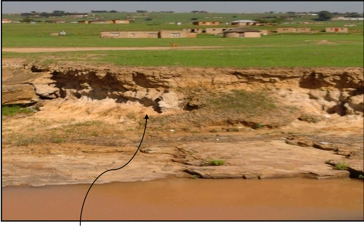
Photo 5: Showing erosion along the river banks.
