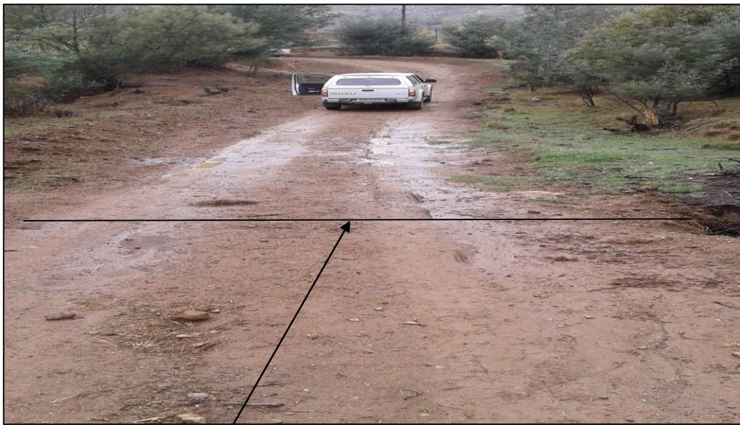
Photo 3: showing the water crossing on the existing track
