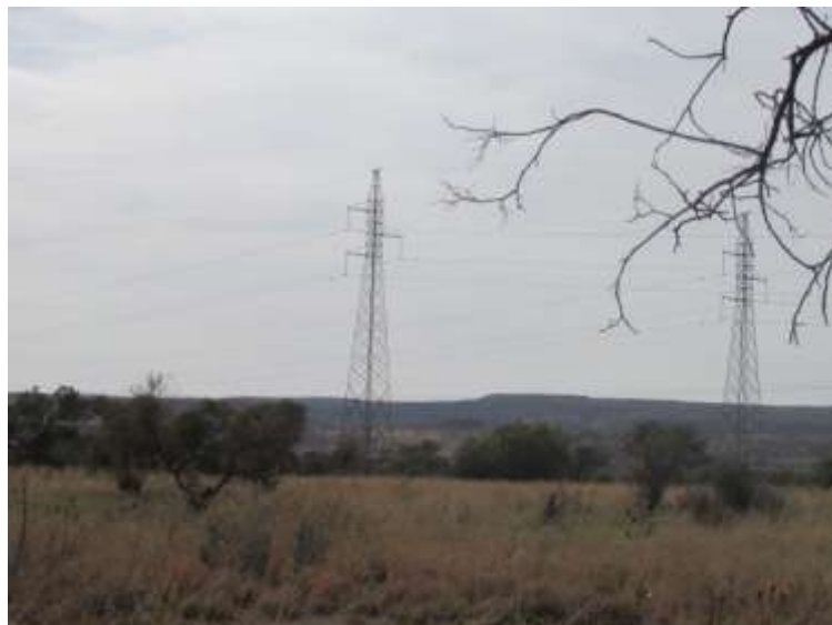
Figure 7: View of the existing ESKOM Lines in the area.
