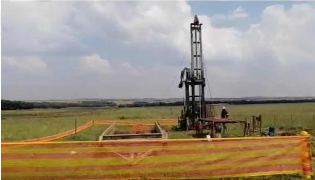
Figure 14: Example of temporary fence
