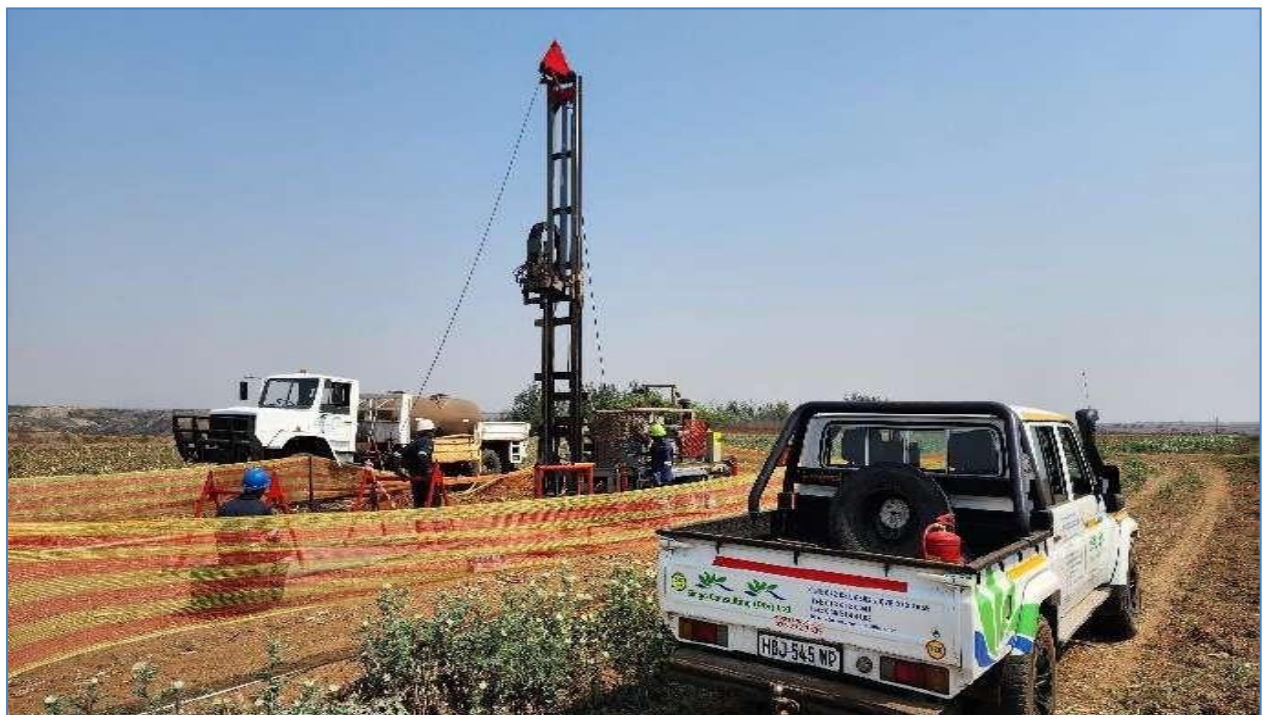
Figure 9: A typical example of a drilling site.
