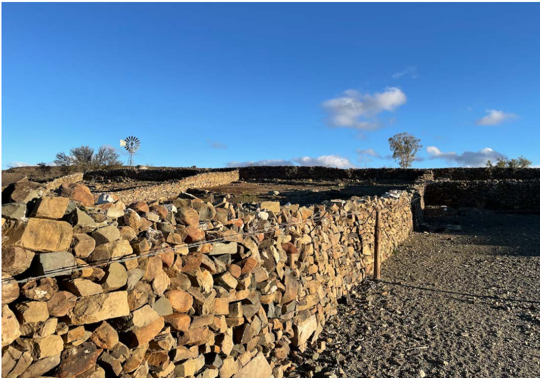
Figure 18: Stone walls at the farmhouse providing roosting opportunities for bats
