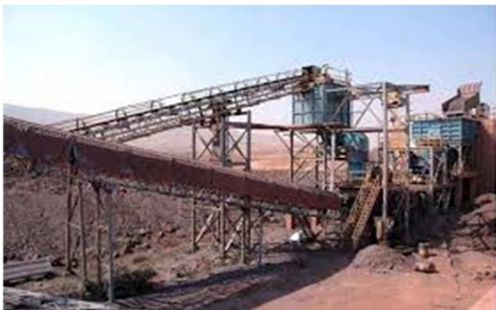
Figure 3 – Typical Crusher and Screening Plant
