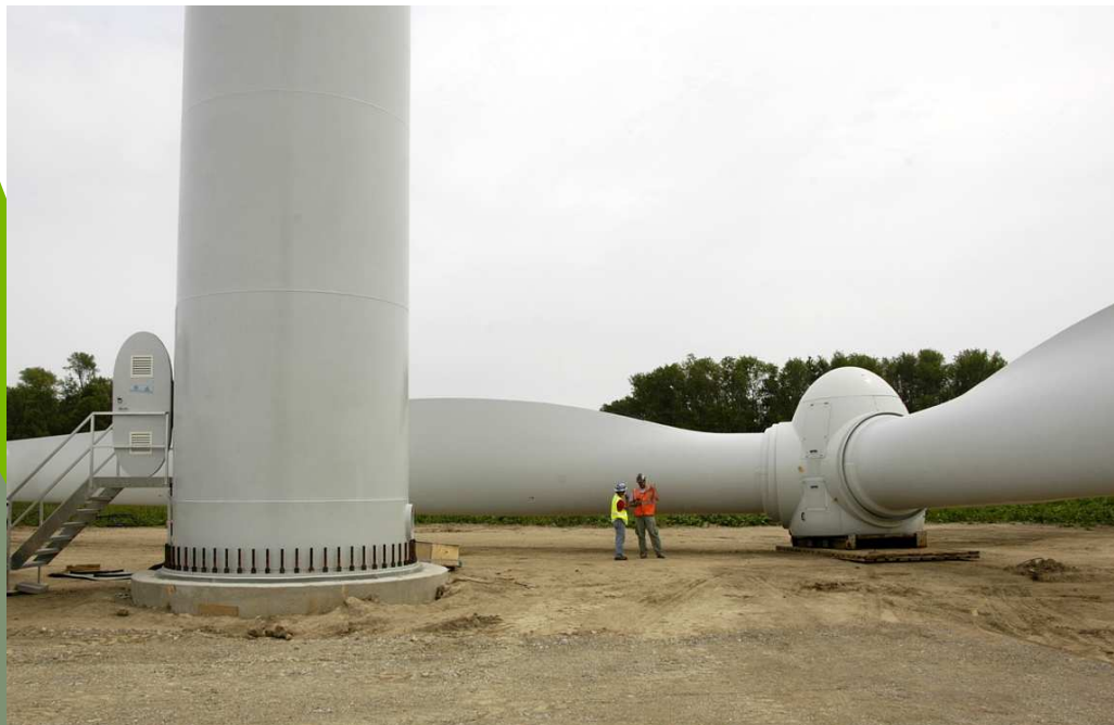
Figure 3 Wind turbine in the process of erection (source http://www.windpowerninja.com/wind-power-government-industry-news/massive-opportunity-for-wind-turbine-production-in-us-66460/ )
