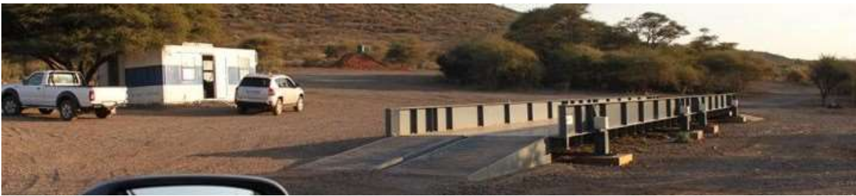
Photo 8: Existing weighbridge and containerised office on site
