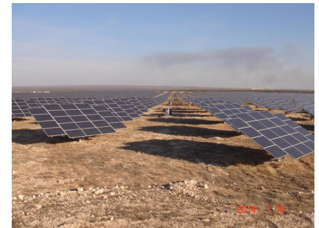
Tracking PV solar panels near Kathu, Northern Cape
