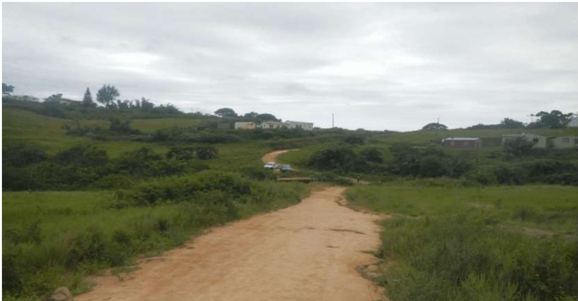
Condition of existing bridge-approaches
