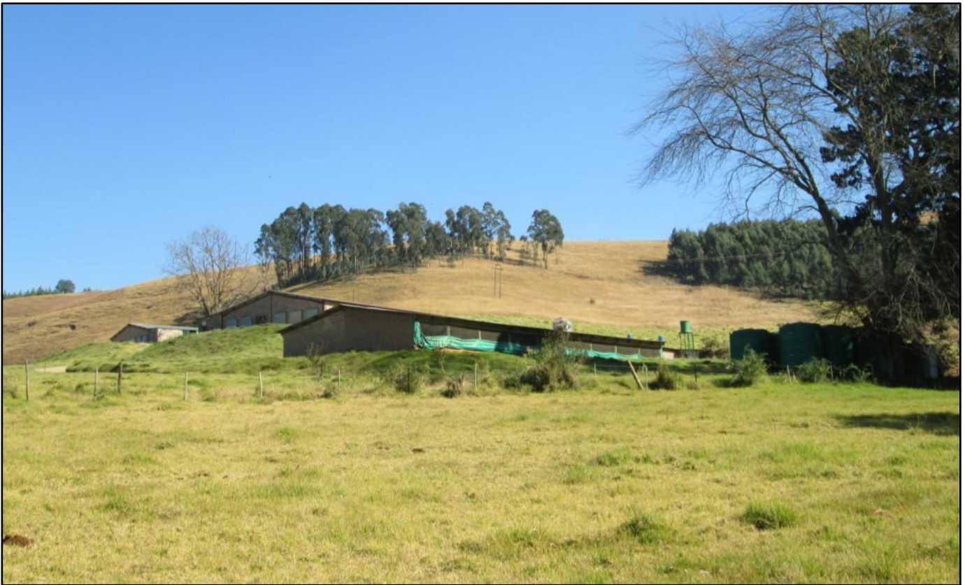
Photo 2: View of the existing rearing houses, located to the west of the proposed new rearing house site.
