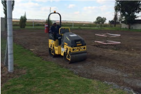
Figure 2: Composting pad preparation
