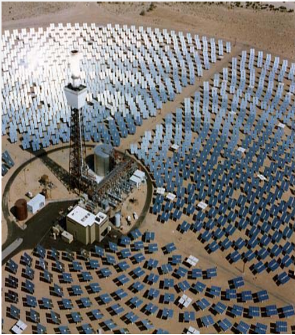
Figure 2: An example of a power plant using central receiver (tower) technology. This is a 10 MW demonstration plant built in the United States – image courtesy of NREL.
