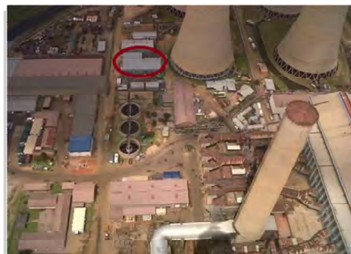
Desalination plant: View of the plant facing east (the L shaped building to the left of the left foreground cooling tower is the main building housing the membranes for the desalination plant, the pumps are in the open to the western side.)
