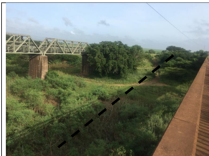
Figure 1. Image looking north showing the proposed alignment of the Mkuze River crossing pipeline bridge.
