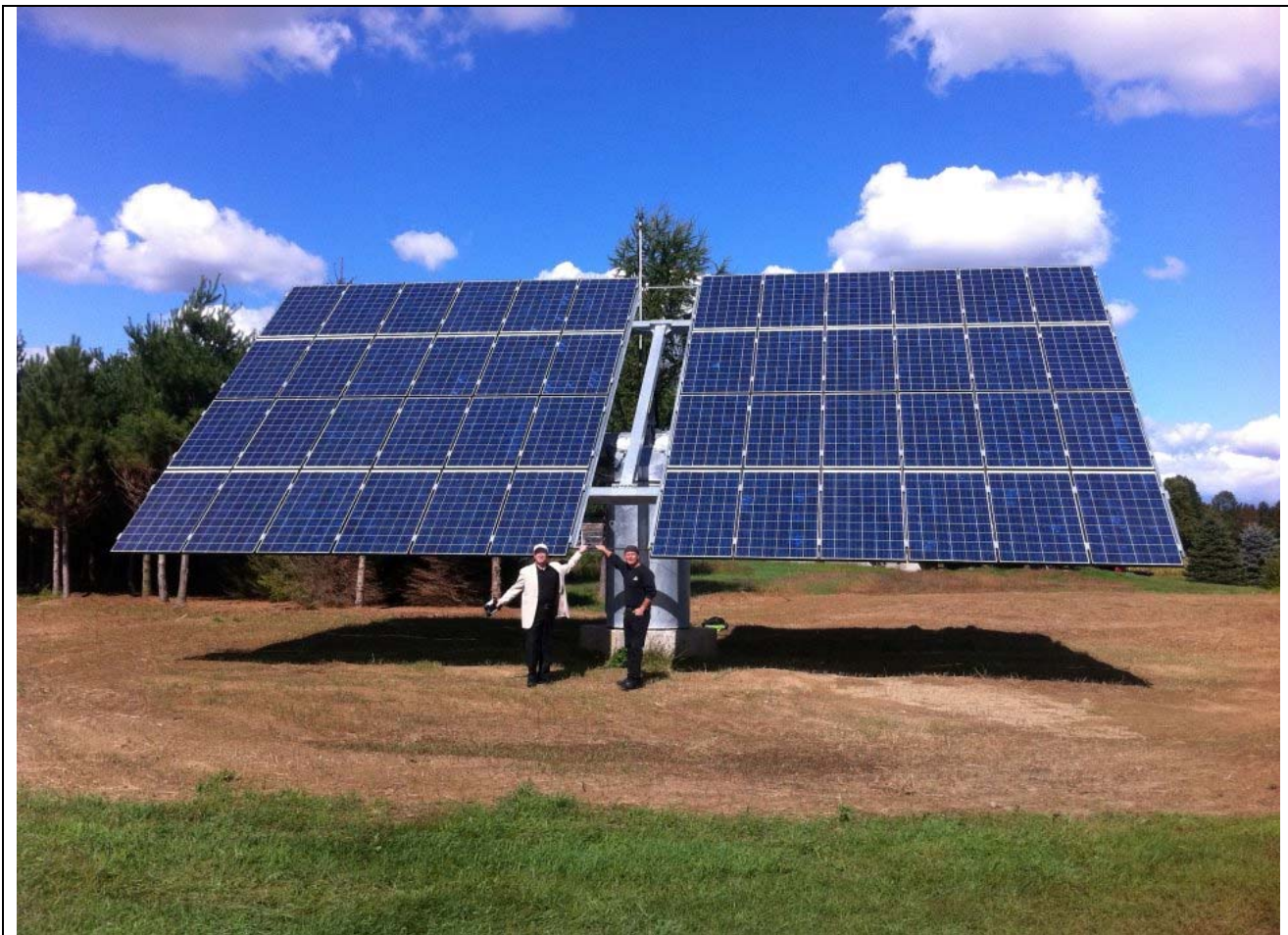
Figure 3-2: Tracking PV array (sourced http://solarblog.ca )
