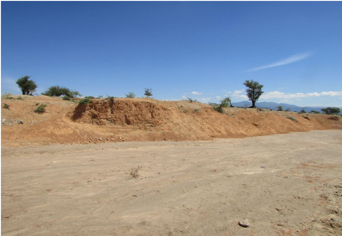
Figure 6: Closer view of the (currently) dry Rapholo Riverbed at the location where the new bridge will be constructed.
