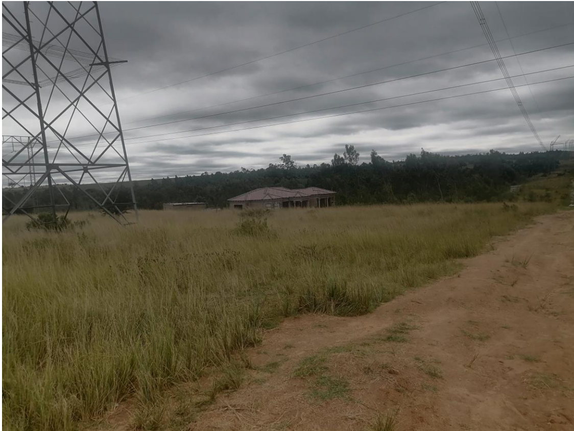
The HV powerline on site
