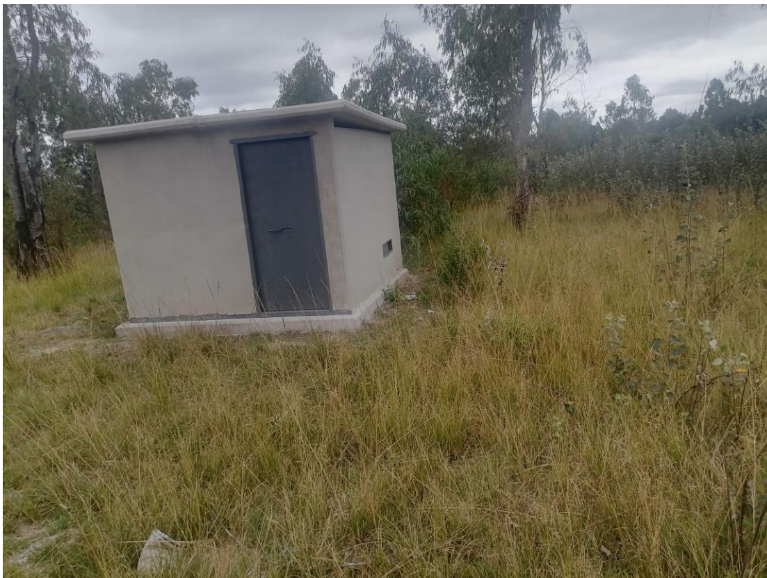
This borehole require electricity
