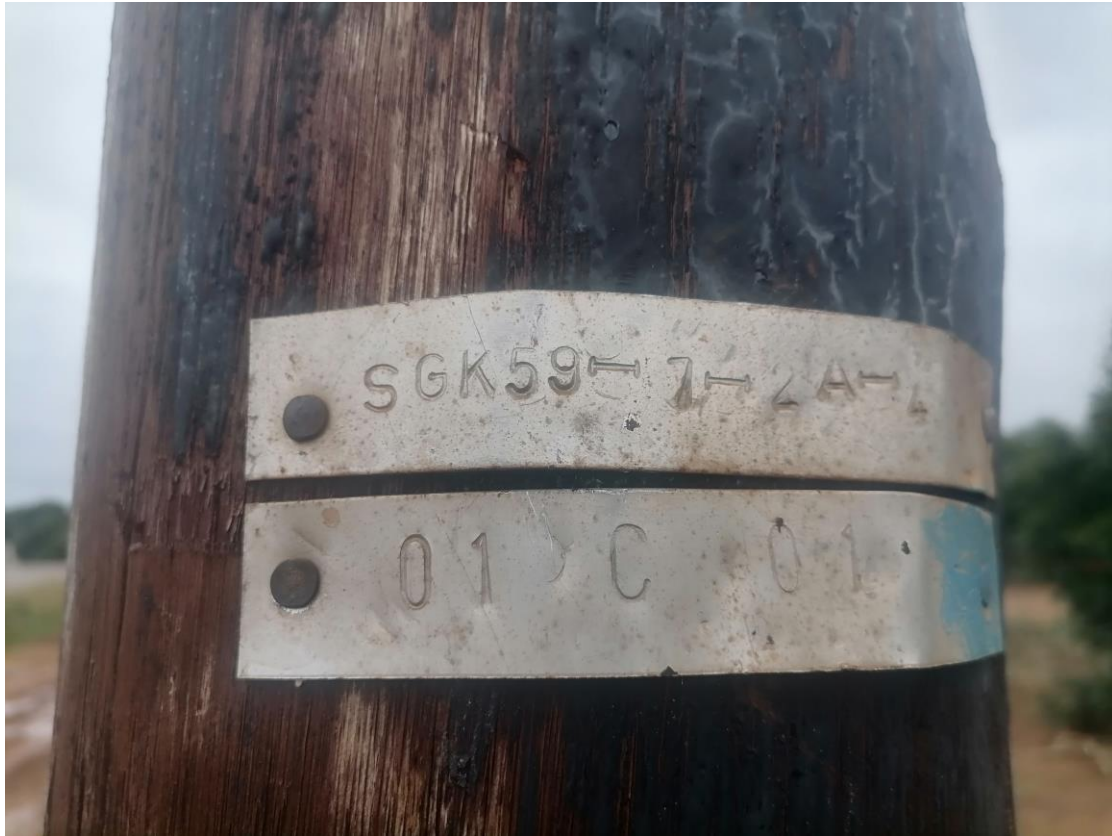
The existing pole number on site
