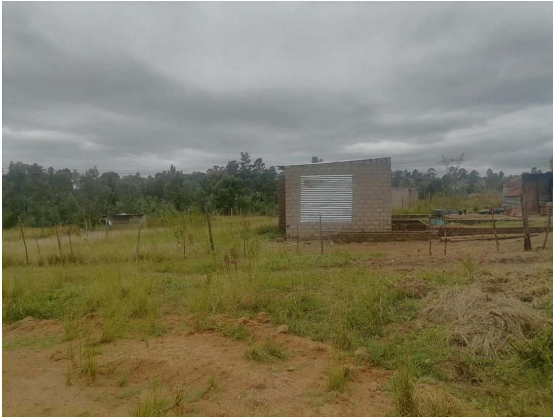
Houses with no electricity
